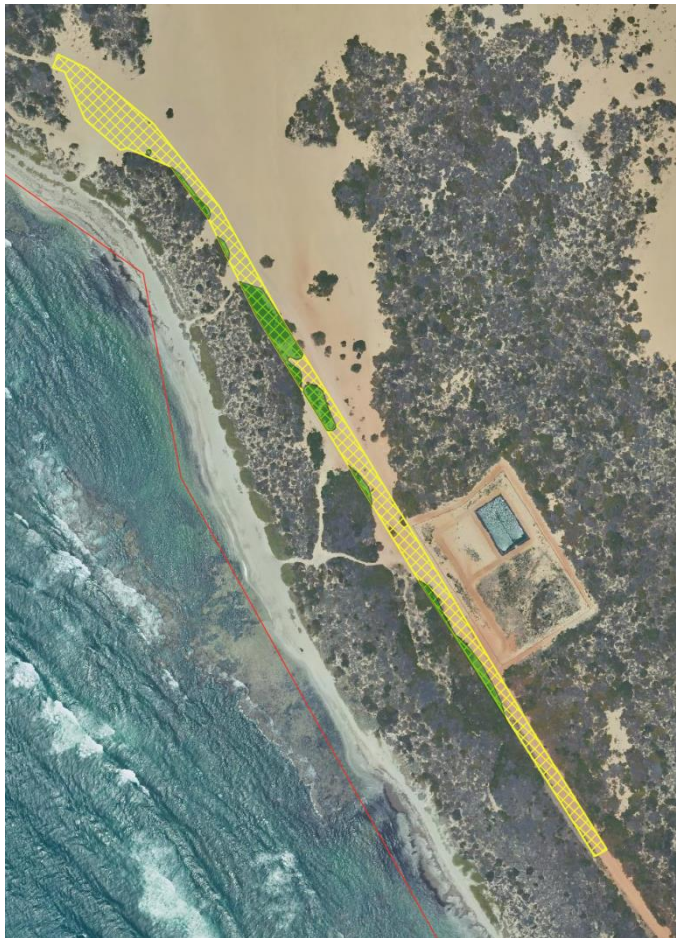
Figure 2: An image representing the area of the actual clearing (green) in comparison the application area footprint (yellow)
