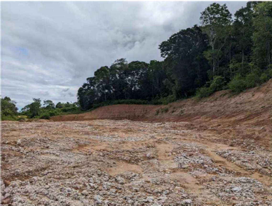
Figure 23: Waypoint 4, looking North.
