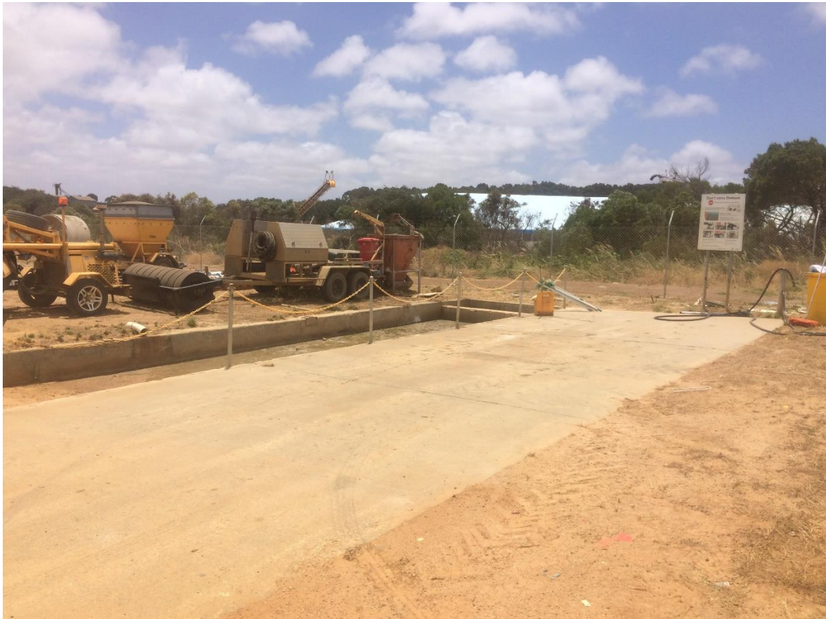
Figure 1. Shire of Esperance Depot vehicle washdown bay
