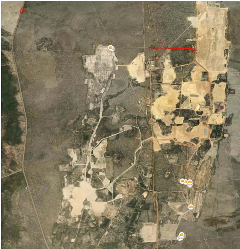
Plate 16: Location of photos of rehabilitation from the 82 Strand and South Tails Location (Plate 1-14). The red areas indicate the area within which conditional authorised clearing can occur under the granted clearing permit.
