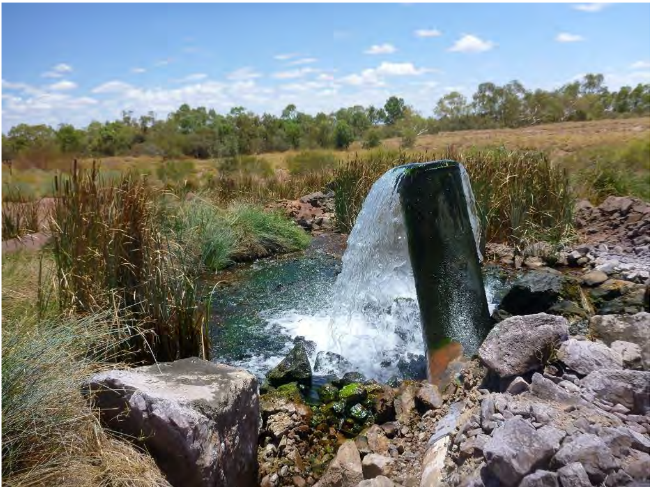
Plate 1-1: The W12 (Topvar) discharge outfall.
