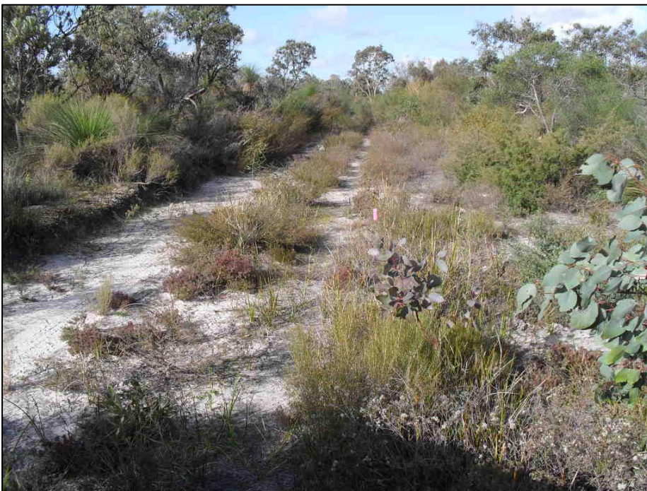
Plate 2. Example of minimal impact drill line. Trees have been avoided, vegetation on the track remains in-situ, minimal topsoil disturbance, track limited to width of standard road vehicle.
