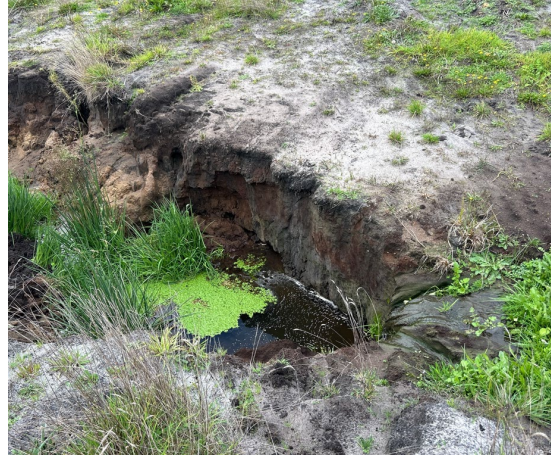
Photo 3-7 Erosion present along drainage line
