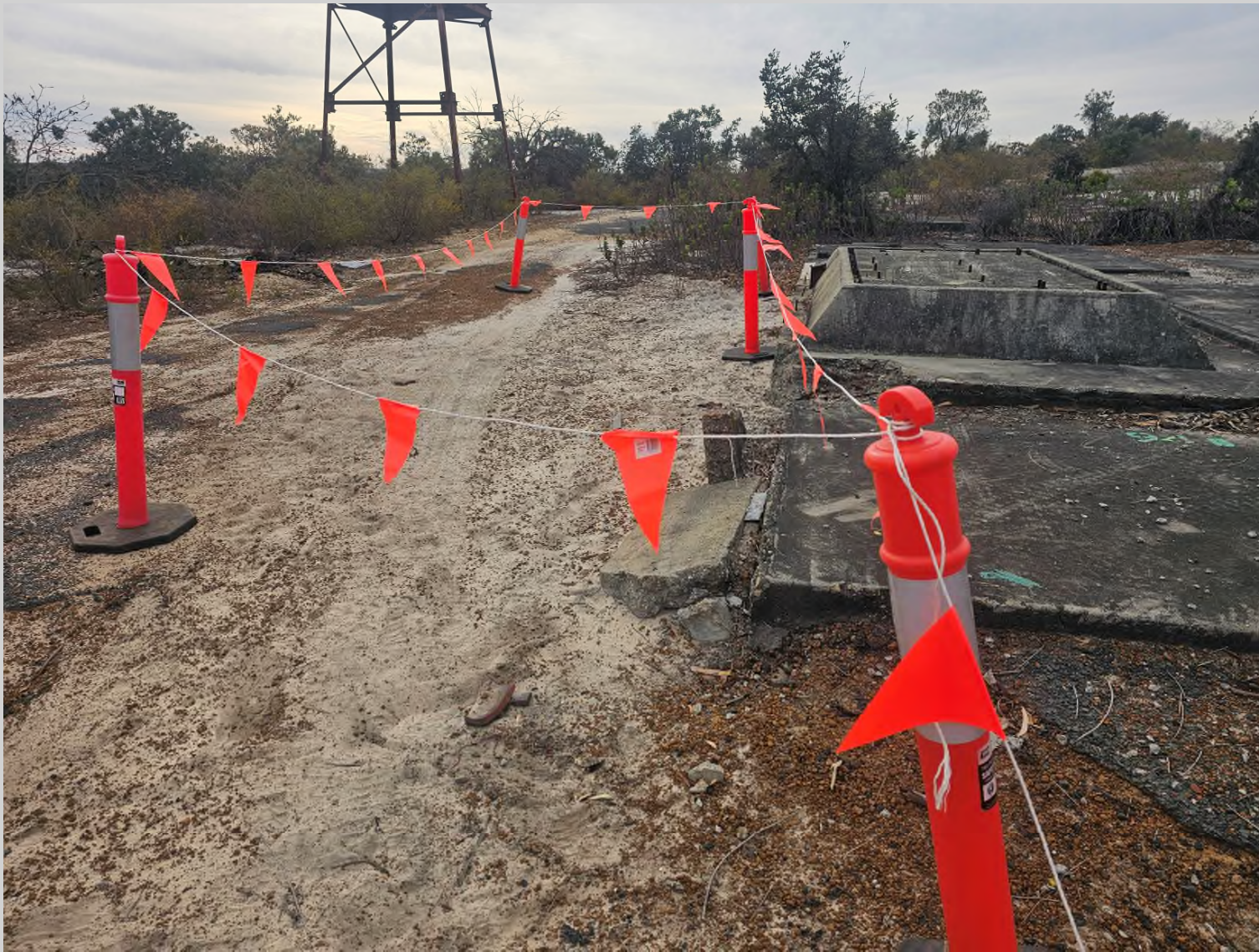
Photo 5 – ACM Impacted Area 1B Looking East
