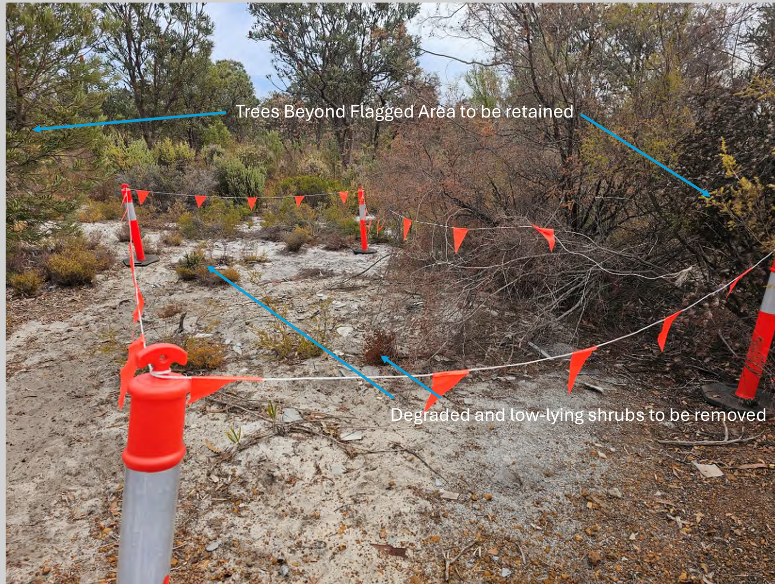
Photo 3 – ACM Impacted Area 6
