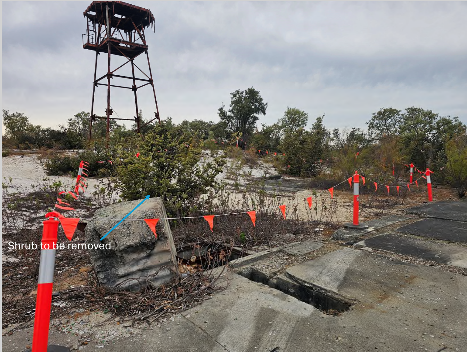
Photo 27 – ACM Impacted Area 1F Looking South
