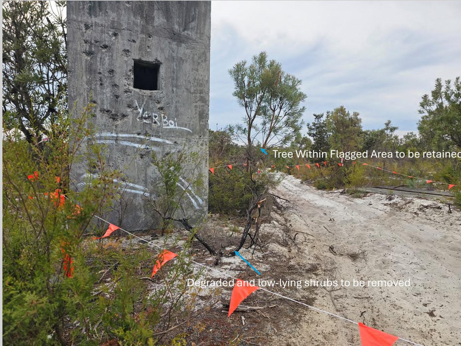
Photo 12 – ACM Impacted Area 7
