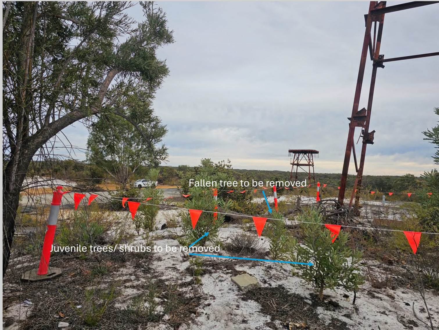
Photo 21 – ACM Impacted Area 1E Looking north towards Area 1C
