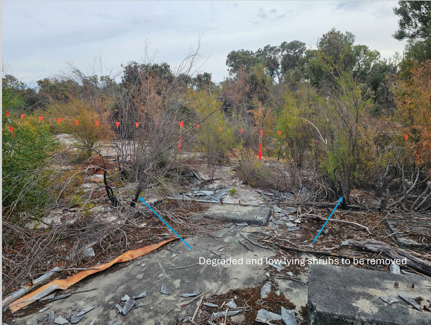
Photo 9 – ACM Impacted Area 2 Looking West
