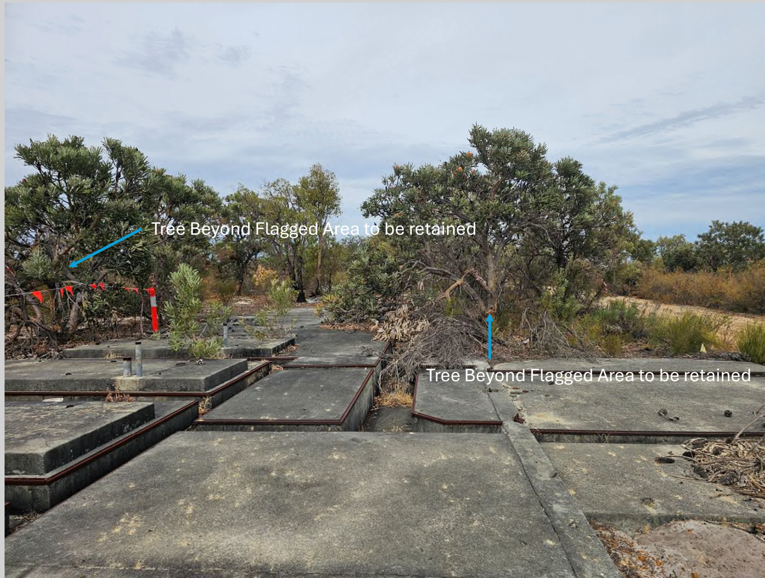
Photo 3 – ACM Impacted Area 3
