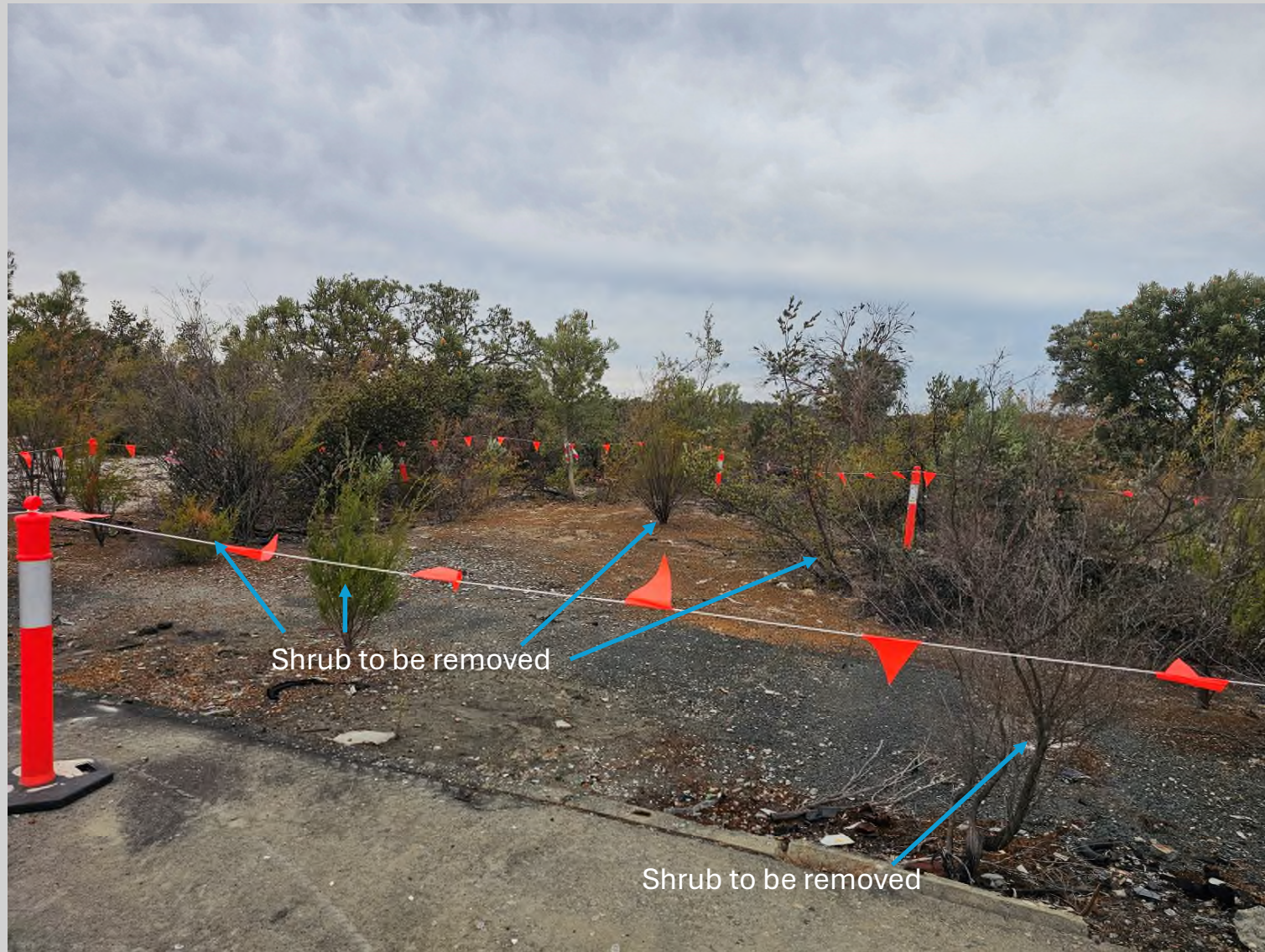
Photo 28 – ACM Impacted Area 1F Looking East
