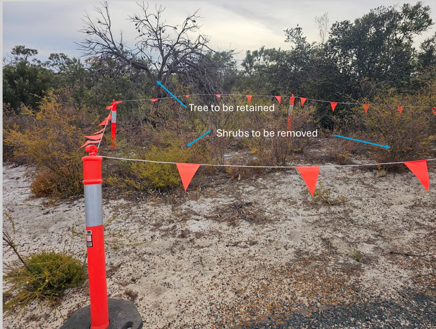
Photo 13 – ACM Impacted Area 1C Looking East From Cleared Track Around Tower
