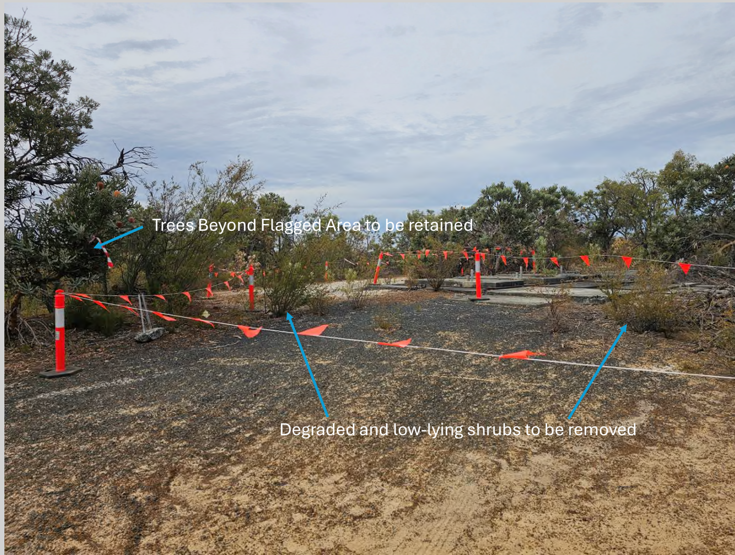
Photo 2 – ACM Impacted Area 3
