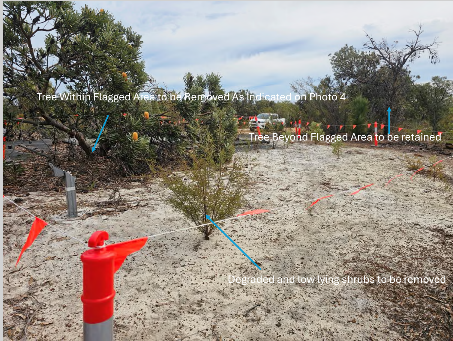
Photo 7 – ACM Impacted Area 3
