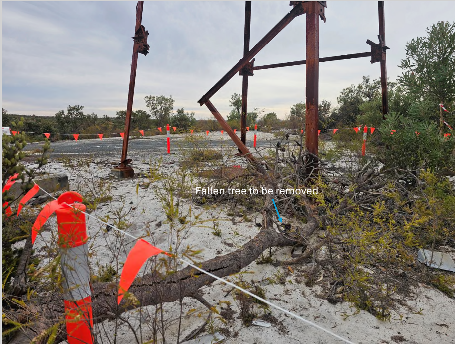
Photo 22 – ACM Impacted Area 1E Looking East
