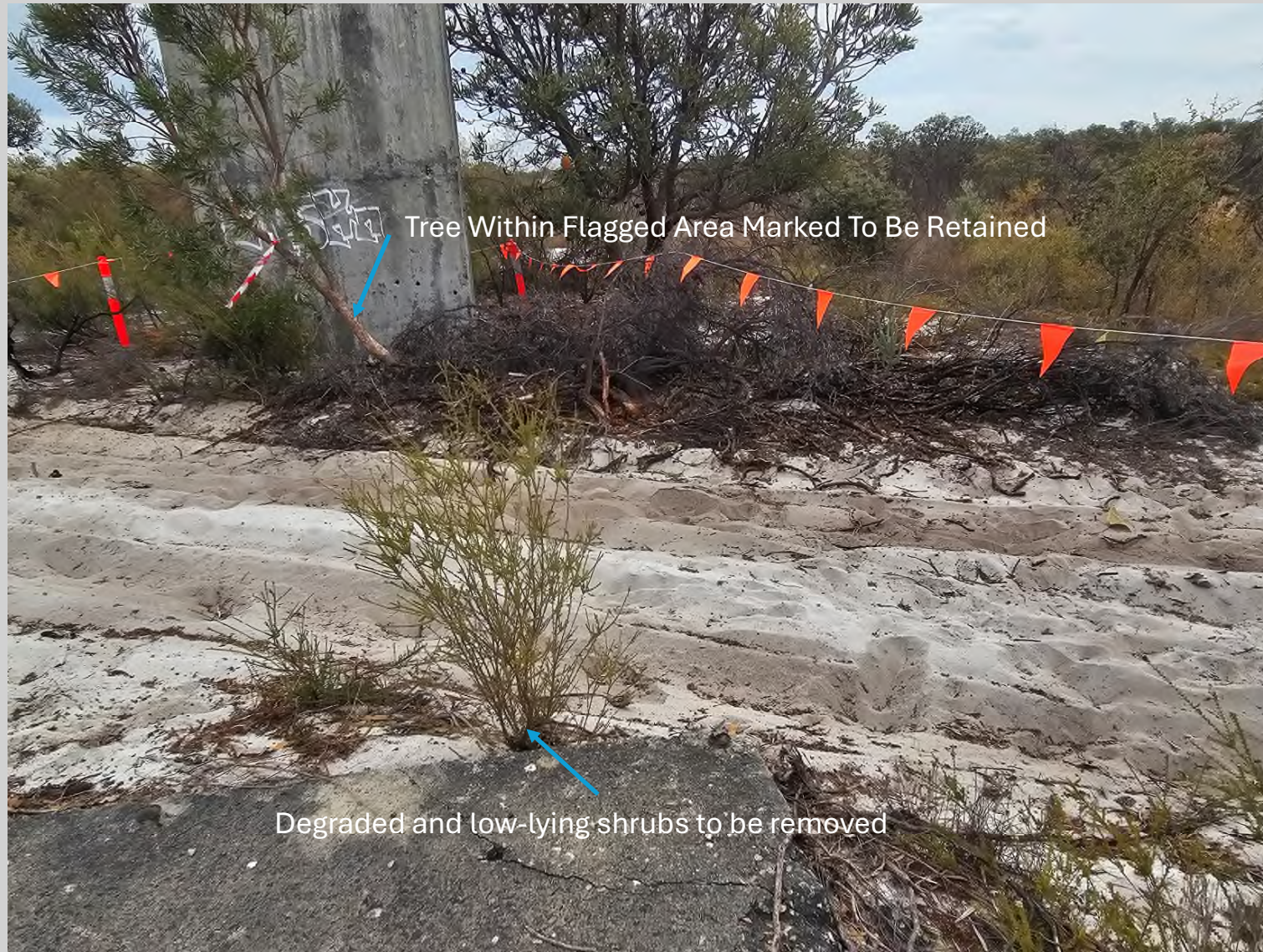
Photo 10 – ACM Impacted Area 7
