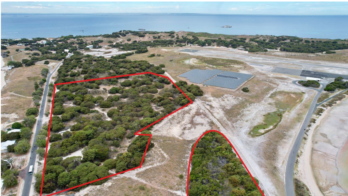
Plate 1: Aerial photograph of the site with indicative clearing area outlined in red
