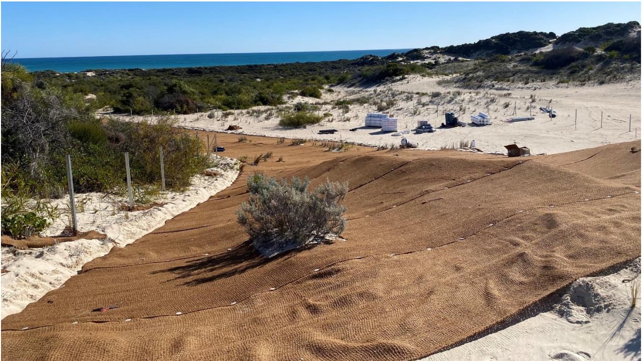
Figure 9: Example of erosion control matting installed by Natural Area at Catalina Foreshore for Tamala Park Regional Council (2023).
