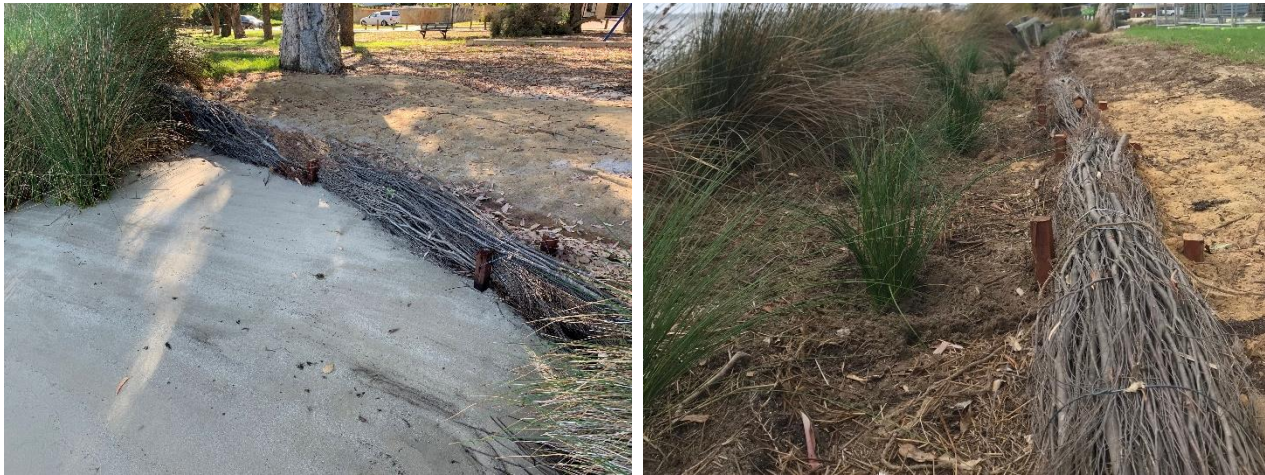
Figure 8: Examples of brush walling performed by Natural Area at various sites, ( left ) Canning Foreshore, ( right ) Melville Beach Foreshore.
