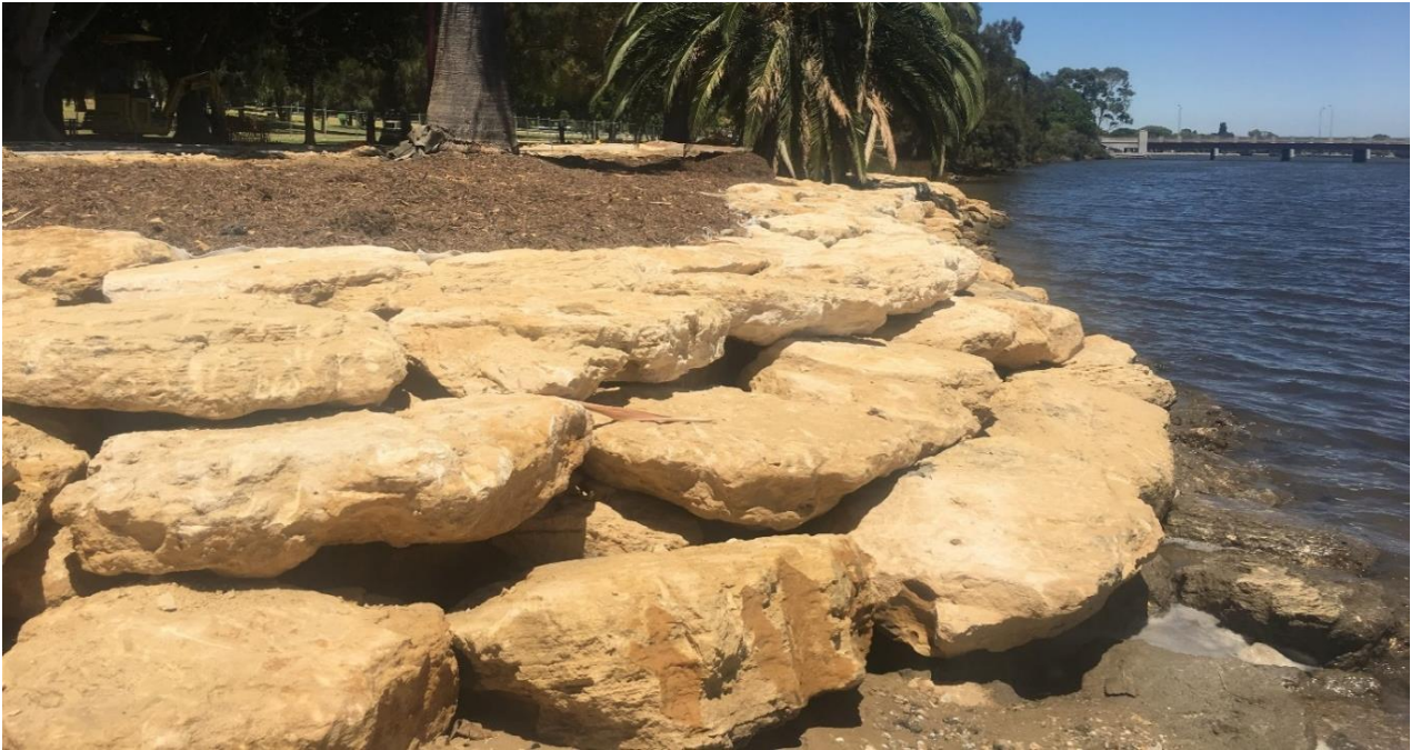
Figure 6: Biscuit rock revetment constructed by Natural Area along the Burswood Foreshore in January 2019.
