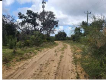
Communication tower and powerlines
