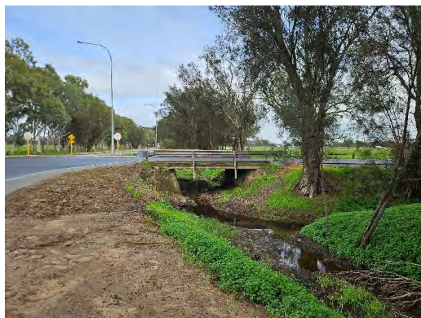
Plate 3-2: Kargotich Road Bridge
