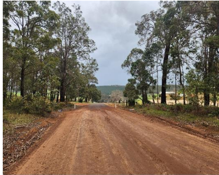
FIGURE 2: ROADSIDE CONDITION- NATURAL AREA
