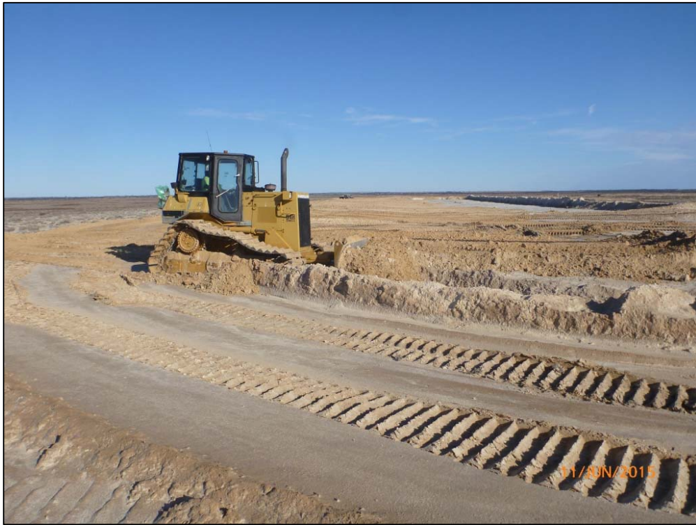
Plate 17: Rehabilitation photo taken 11/06/2015 at M70/1191
