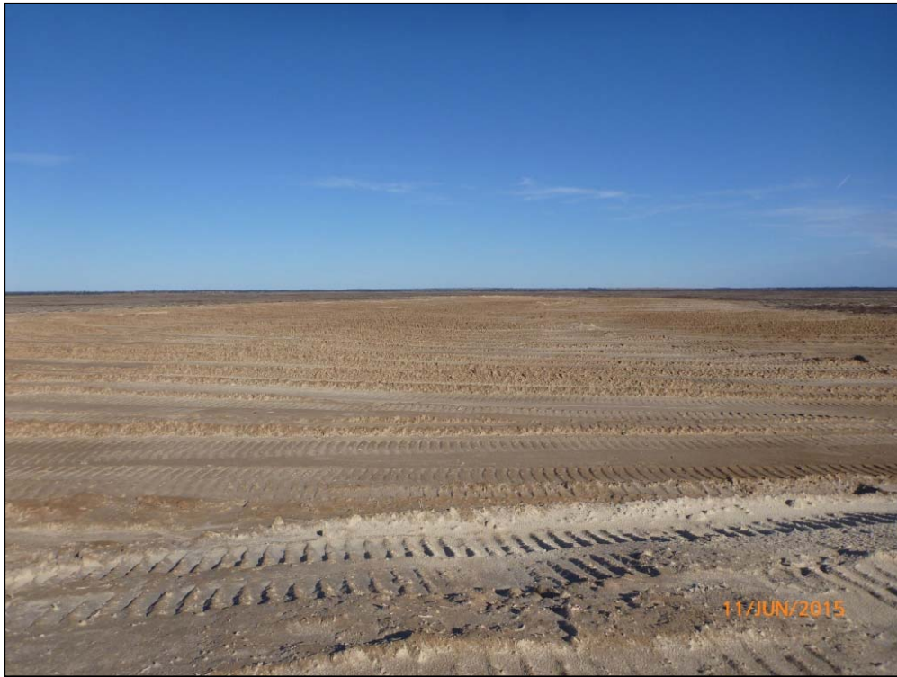
Plate 21: Monitoring Site 7 in 2015 (immediately after rehabilitation earthworks)
