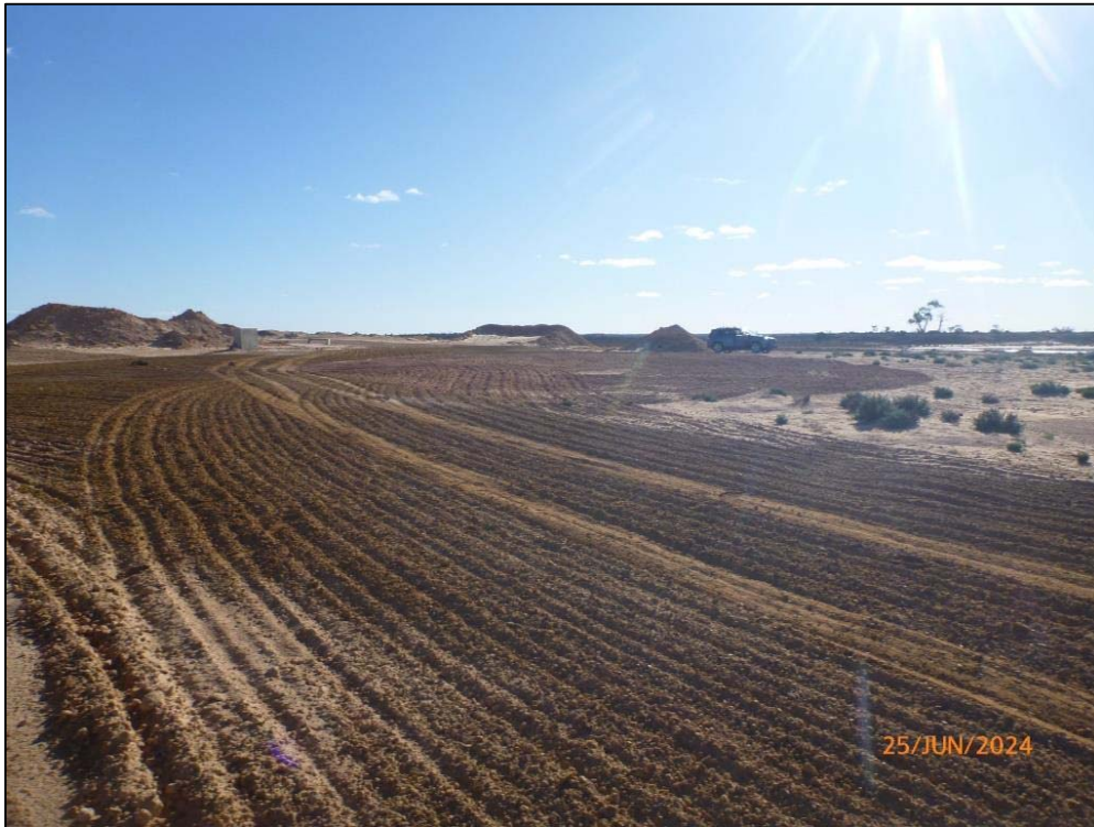
Plate 36: Ripped access roads to mined-out areas on M70/1079
