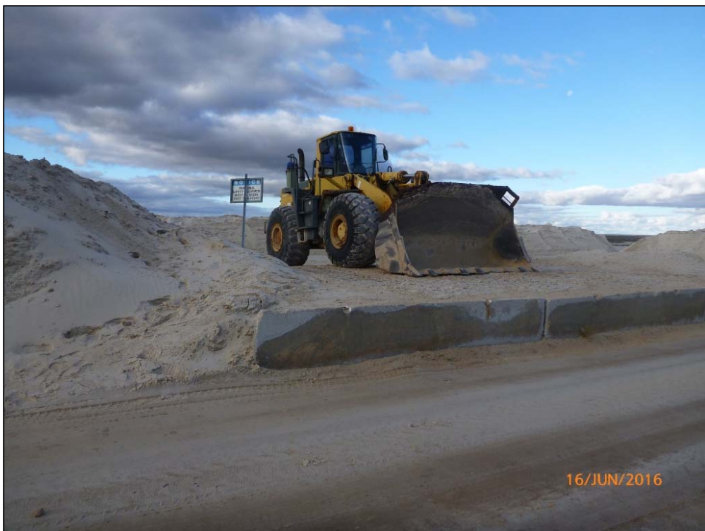
Plate 10: Load-out at the stockpiling area on M70/1118
