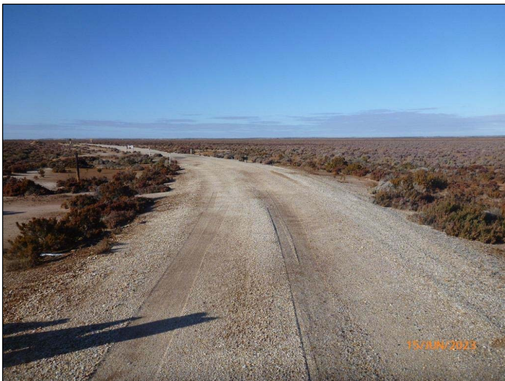
Plate 8: Access road on L70/72, looking towards the stockpiling area on M70/1118
