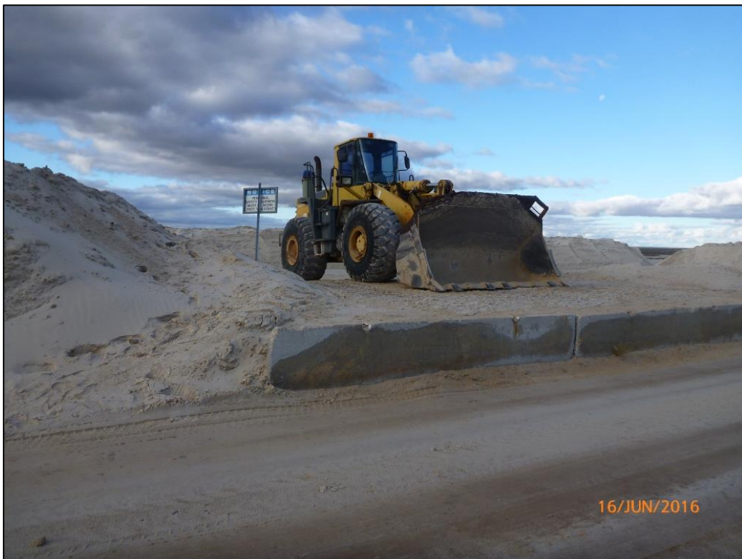
Plate 8: Load-out at the stockpiling area on M70/1118
