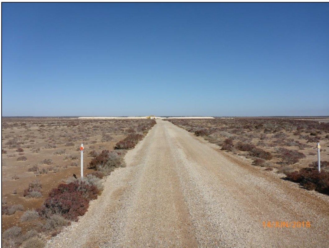
Plate 6: Access road on L70/72, looking towards the stockpiling area on M70/1118
