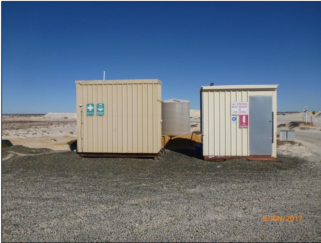
Plate 11: Site office and ablution block on M70/1255
