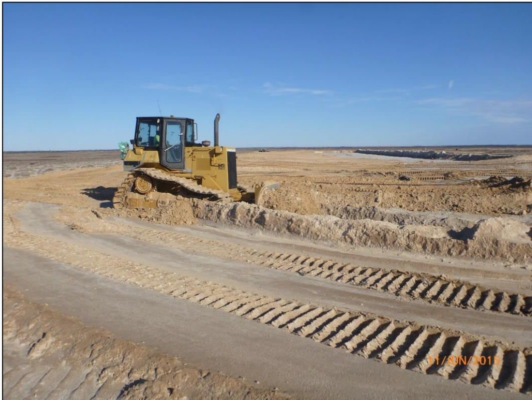
Plate 15: Rehabilitation photo taken 11/06/2015 at M70/1191
