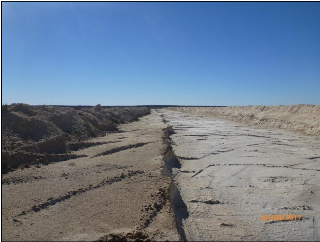
Plate 13: Mining area on M70/1118 showing resource depth
