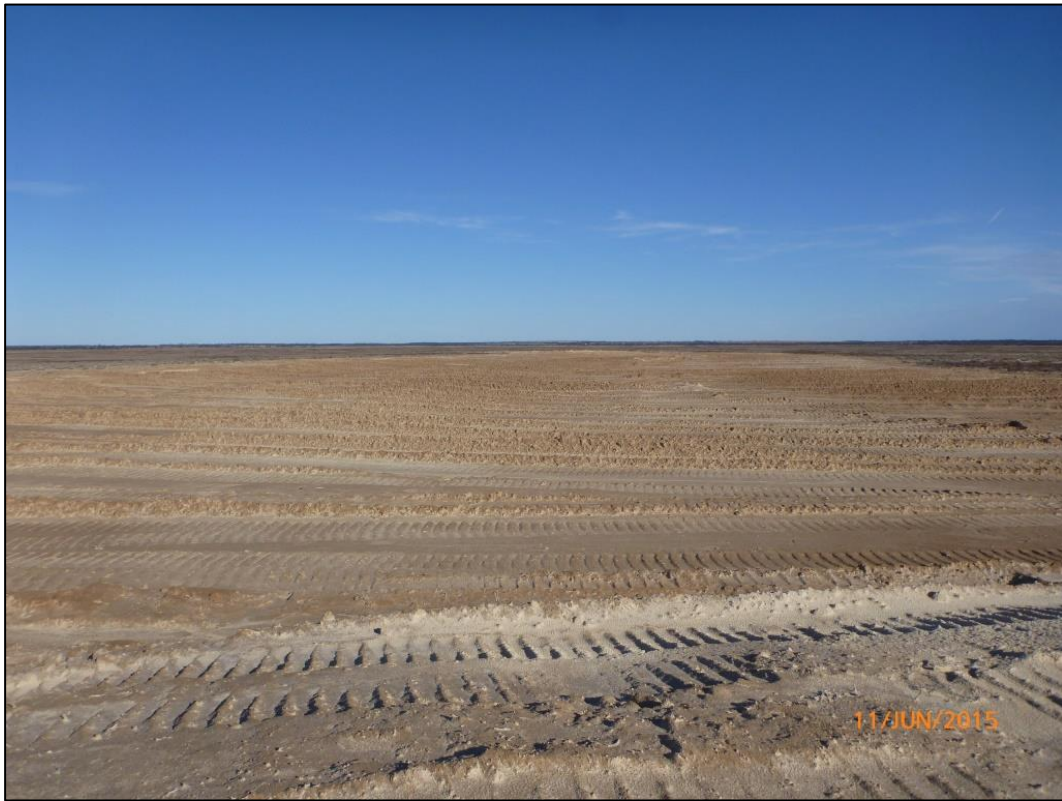
Plate 19: Monitoring Site 7 in 2015 (immediately after rehabilitation earthworks)
