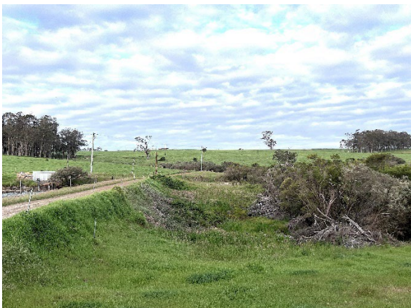
Photo 5. Waterlogged area adjacent to dam wall; Site 2.
