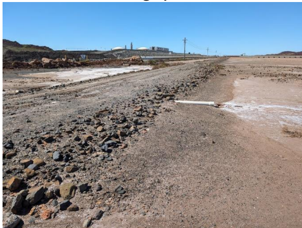
[04 Jul 2024] – Drainage line discharging north of the site.
