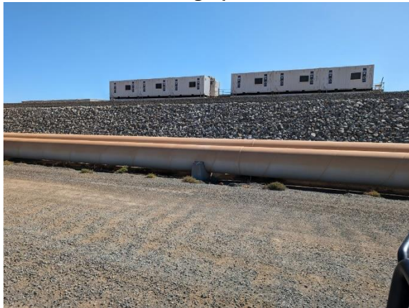
[04 Jul 2024] – Water pipeline north of the site
