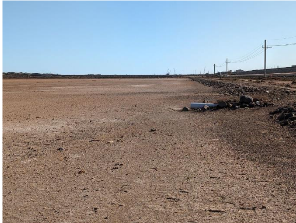
[04 Jul 2024] – Site conditions, looking west
