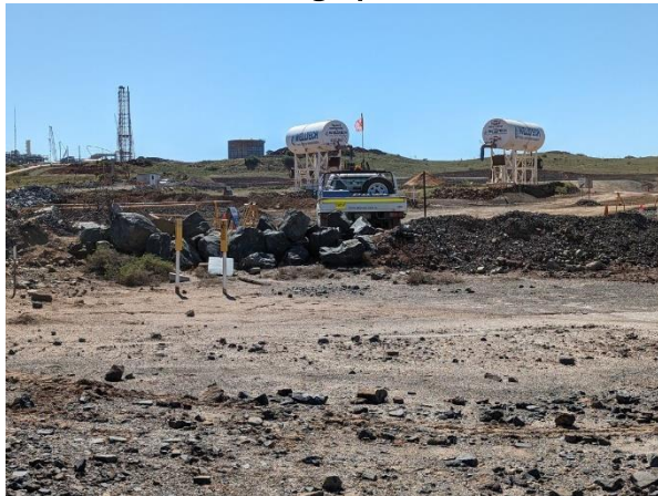
[04 Jul 2024] – Active works area northwest of the site.
