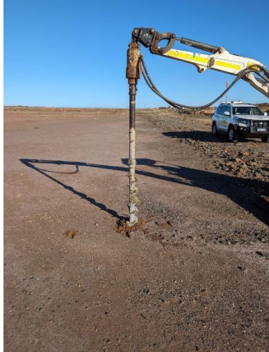
[04 Jul 2024] – Monitoring well installation (MW02)
