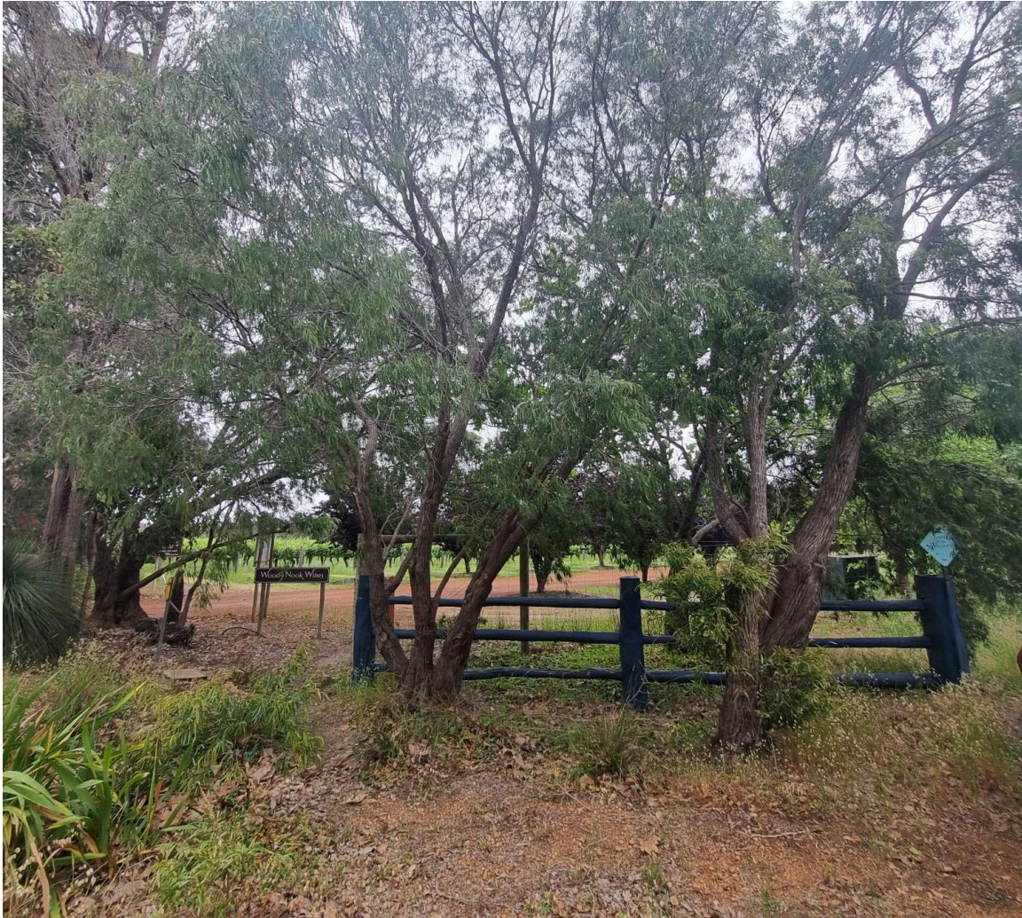
Photo 3: Northern side of Metricup Road (looking north). Clearing required for power pole (a 'structure' and therefore subject to exemption). Two mature Agonis flexuosa trees will be cleared (115.08065843, -33.78178329).
