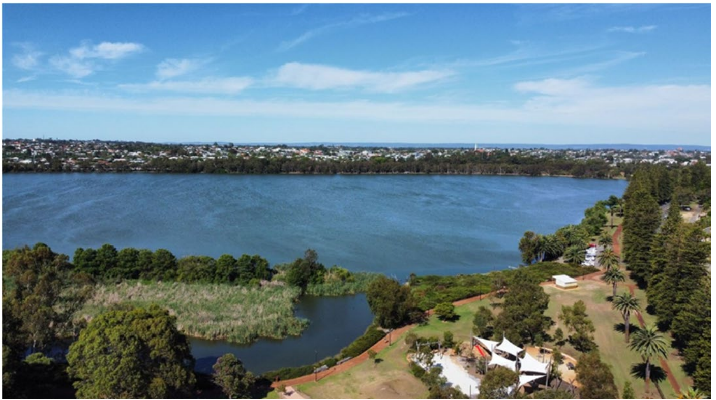
Below: Drone view of site
