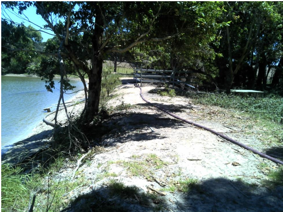
Photopoint 7: Top of dam wall
