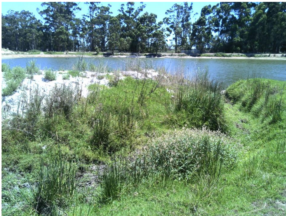
Photopoint 5: Looking north showing existing dam wall
