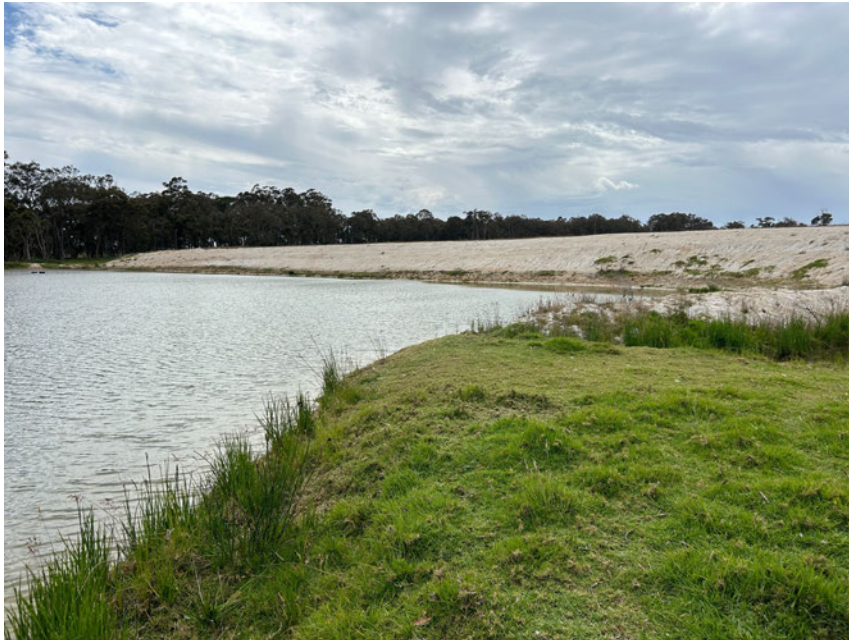
Plate 4a: Dam wall from south-west side looking east.
