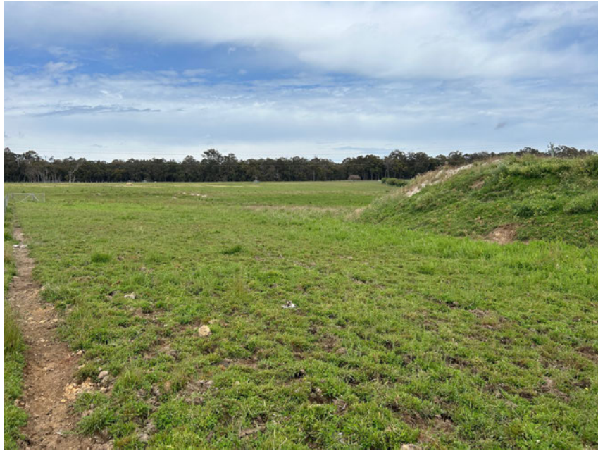
Plate 3: Paddock adjacent dam wall.
