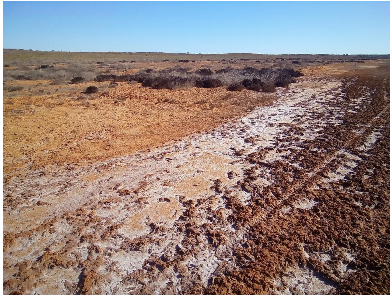
Plate 2 Degraded roadside vegetation
