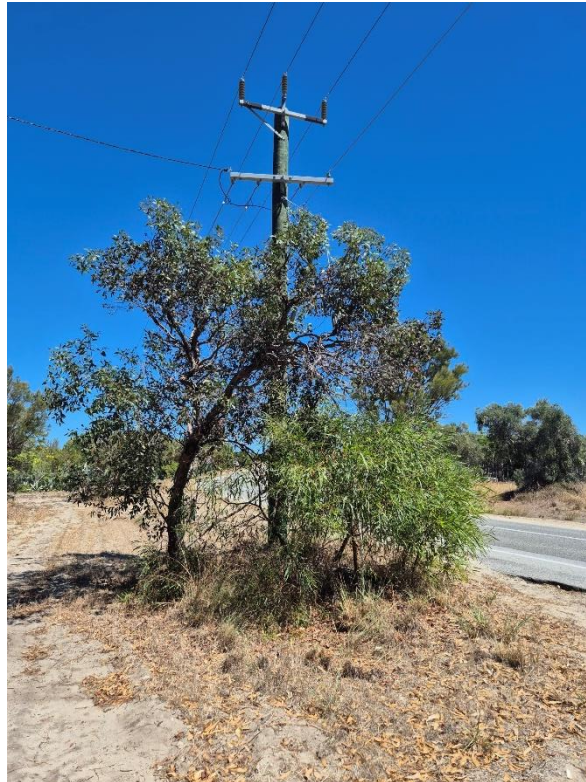
Trees at the base of the power poles with dry litter at the base.
