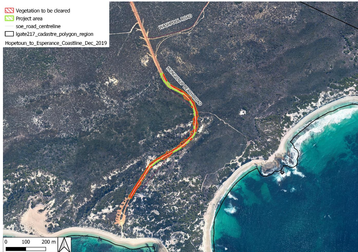
Figure 1. Location of Munglinup Beach Road project.
