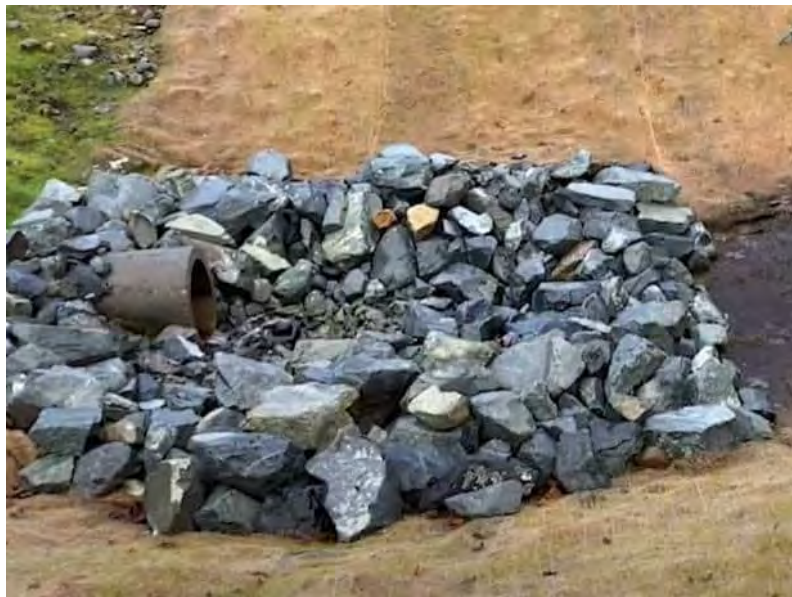
Plate 1 Gravel Lined Outfall/ Channel
