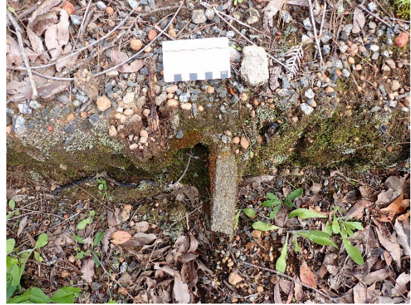
Plate 21. Pipe coming out of the wall set back into the hill slope
