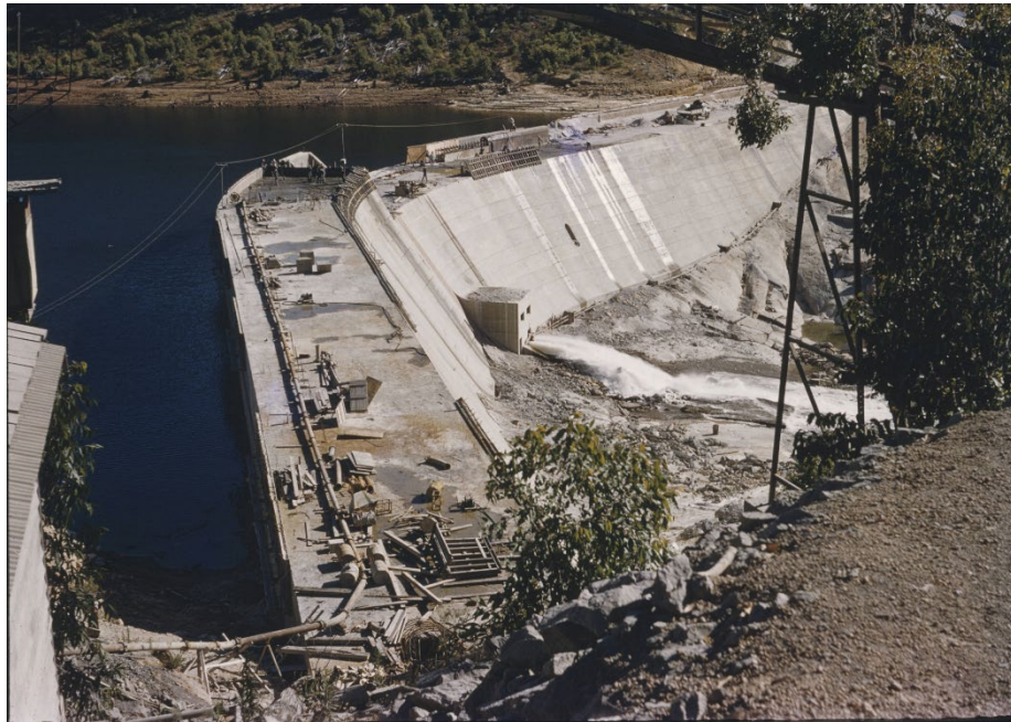
Figure 6. Raising the wall of Wellington Dam, 1960 (photo courtesy of SLWA: 140247PD)
