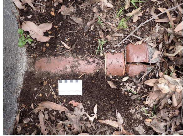
Plate 47. Earthenware pipe at the base of the water tower
