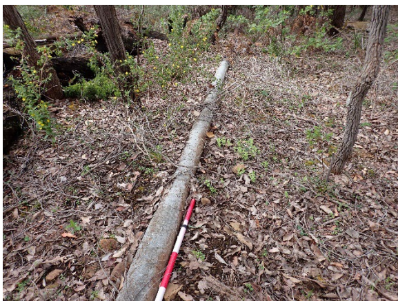
Plate 64. Galvanised steel drainage pipe
