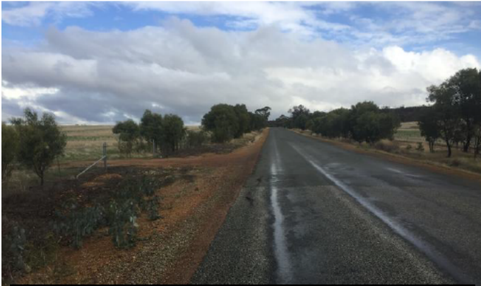
Photo of Pavement Failure on the Pingelly / Alderside Rd at SLK 4.61 due to no adequate table drain and / or lack of maintenance. This pavement failure is the result of no crossover pipe to convey surface water under the crossing and this water has penetrated the underlying soil, resulting in this pavement failure downstream.
