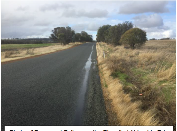
Photo of Pavement Failure on the Pingelly / Alderside Rd at SLK 3.89 due to non-adequate table drainage and / or subsequent lack of maintenance.
