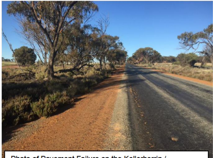
Photo of Pavement Failure on the Kellerberrin / Bencubbin Rd at SLK 16.69 due to non-adequate table drainage and / or subsequent lack of maintenance.
