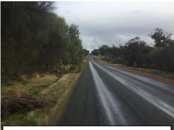
Photo of Pavement Failure on the Pingelly / Alderside Rd at SLK 4.61 due to non-adequate table drainage and / or subsequent lack of maintenance.
