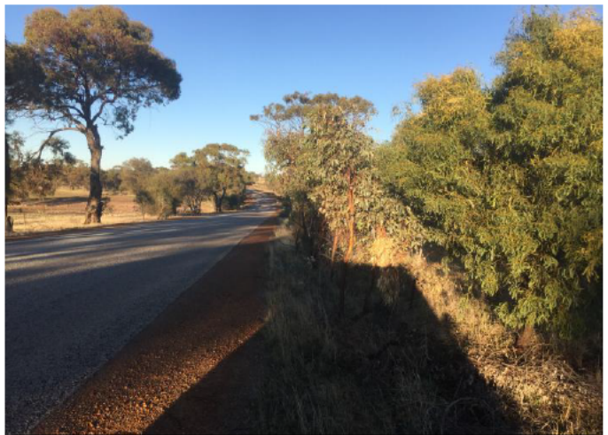
Photo of poorly maintained table drain on the Kellerberrin / Yoting Rd at SLK 17.58 due to insufficient table drain width to allow easy maintenance via Grader. Note this pavement has been upgraded relatively recently and has not had sufficient time to develop potential failure areas.
