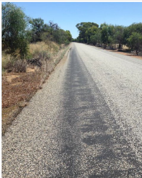
Photo of Pavement Failure on the Goomalling / Calingiri Rd at SLK 24.78 due to non-adequate table drainage and / or subsequent lack of maintenance.
