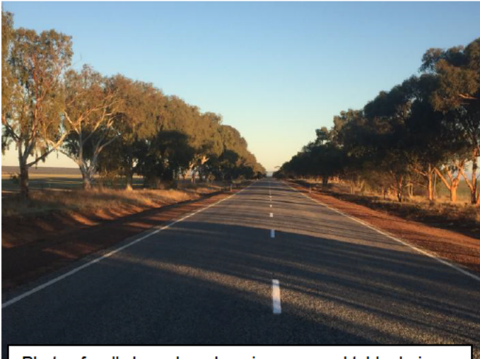
Photo of well shaped road carriageway and table drains on the York / Merredin Rd (MRWA controlled Highway) at SLK 83.66 with well maintained (via Grader) table drains.
