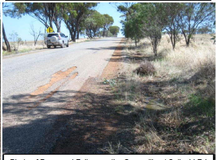
Photo of Pavement Failure on the Goomalling / Calingiri Rd at SLK 11.64 due to non-adequate table drainage and / or subsequent lack of maintenance. Note the surface water sitting in the drain.
