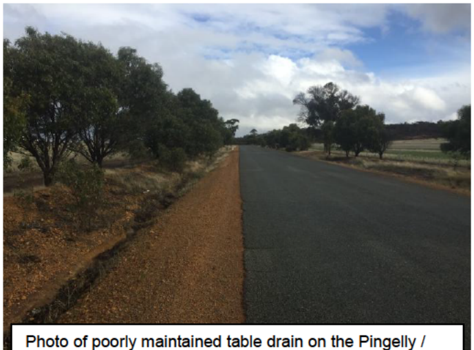
Photo of Pavement Failure on the Pingelly / Alderside Rd at SLK 3.89 due to non-adequate table drainage and / or subsequent lack of maintenance.
