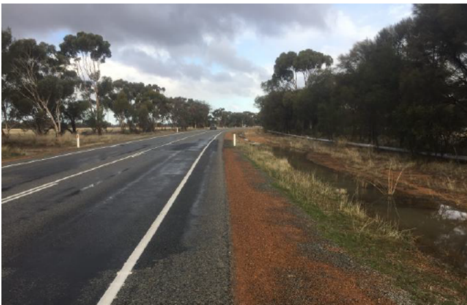
Photo of Pavement Failure on the Great Southern Highway (MRWA Controlled Rd) at SLK 143.20 due to ponding of surface water from no downstream drainage to run water away from pavement (above ground water main has hindered either proper downstream drain construction or limited maintenance of).
