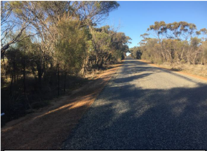
Photo of Pavement Failure on the Kellerberrin / Bencubbin Rd at SLK 13.48 due to non-adequate table drainage and / or subsequent lack of maintenance.
