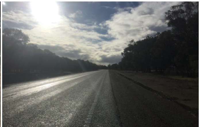
Photo of well shaped road carriageway and table drains on the Great Southern Highway (MRWA controlled Highway) at SLK 148.30 with well maintained (via Grader) table drains. Note the shedding of surface water along the table drain following a large rain event.
