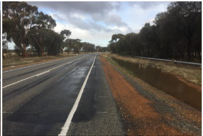
Photo of Pavement Failure on the Great Southern Highway (MRWA Controlled Rd) at SLK 143.15 due to ponding of surface water from no downstream drainage to run water away from pavement (above ground water main has hindered either proper downstream drain construction or limited maintenance of).
