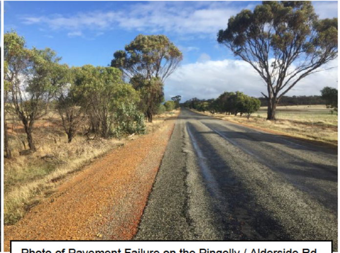
Photo of Pavement Failure on the Pingelly / Alderside Rd at SLK 8.73 due to non-adequate table drainage and / or subsequent lack of maintenance.
