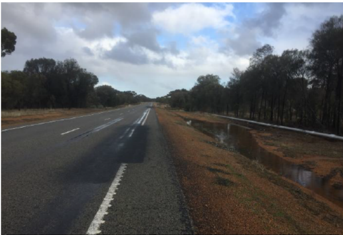
Photo of Pavement Failure on the Great Southern Highway (MRWA Controlled Rd) at SLK 142.53 due to ponding of surface water from no downstream drainage to run water away from pavement (above ground water main has hindered either proper downstream drain construction or limited maintenance of).
