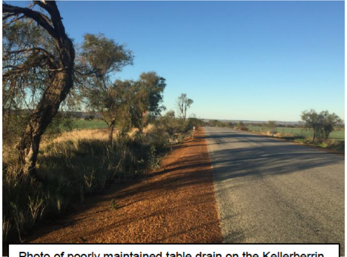
Photo of poorly maintained table drain on the Kellerberrin / Yoting Rd at SLK 20.27 due to insufficient table drain width to allow easy maintenance via Grader. Note this pavement has been upgraded relatively recently and has not had sufficient time to develop potential failure areas.
