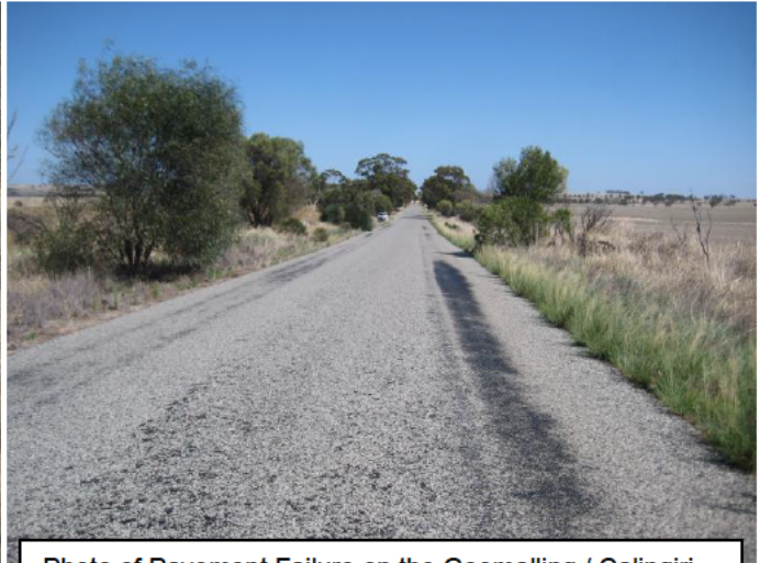
Photo of Pavement Failure on the Goomalling / Calingiri Rd at SLK 6.76 due to non-adequate table drainage and / or subsequent lack of maintenance.
