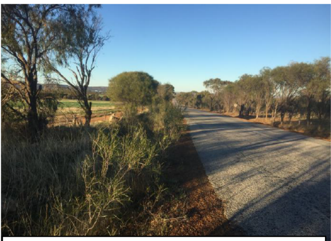
Photo of poorly maintained table drain on the Kellerberrin / Yoting Rd at SLK 19.63 due to insufficient table drain width to allow easy maintenance via Grader. Note this pavement has been upgraded relatively recently and has not had sufficient time to develop potential failure areas.
