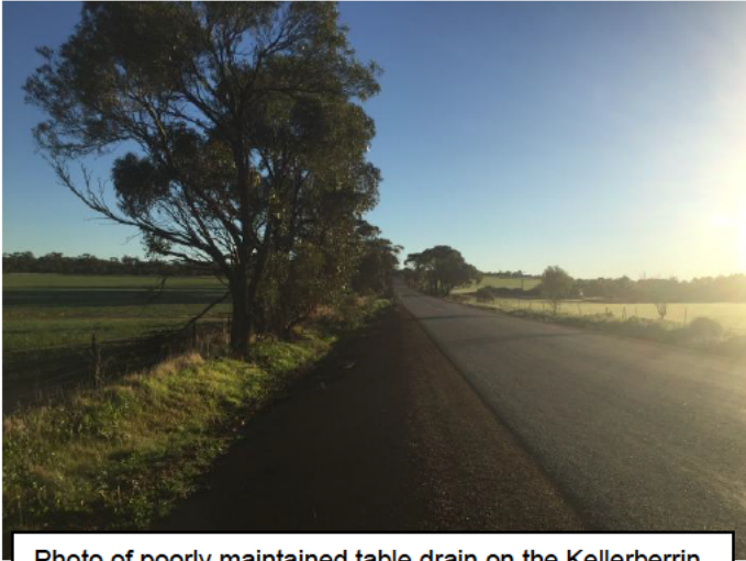
Photo of poorly maintained table drain on the Kellerberrin / Yoting Rd at SLK 20.18 due to insufficient table drain width to allow easy maintenance via Grader. Note this pavement has been upgraded relatively recently and has not had sufficient time to develop potential failure areas.
