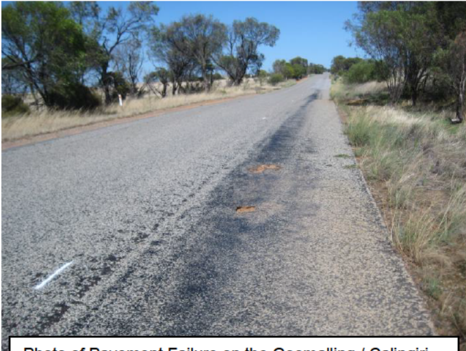
Photo of Pavement Failure on the Goomalling / Calingiri Rd at SLK 5.10 due to non-adequate table drainage and / or subsequent lack of maintenance.
