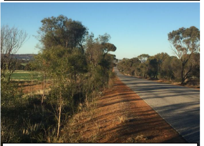
Photo of poorly maintained table drain on the Kellerberrin / Yoting Rd at SLK 19.66 due to insufficient table drain width to allow easy maintenance via Grader. Note this pavement has been upgraded relatively recently and has not had sufficient time to develop potential failure areas.
