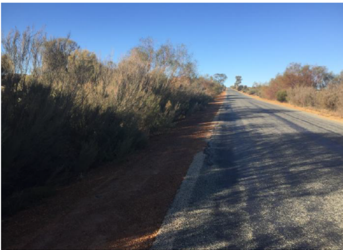
Photo of Pavement Failure on the Kellerberrin / Bencubbin Rd at SLK 22.37 due to non-adequate table drainage and / or subsequent lack of maintenance.
