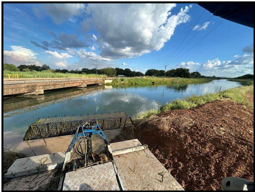
Figure 7: Before the clearing of weeds in channel - minimal disturbance to before and after of the channel bank with minimal sedimentation and erosion to the foreshore area. Also notice the selective removal of the weeds, keeping vegetation along the foreshore areas to ensure bank stability (Hydroscape Environmental, 2025).
