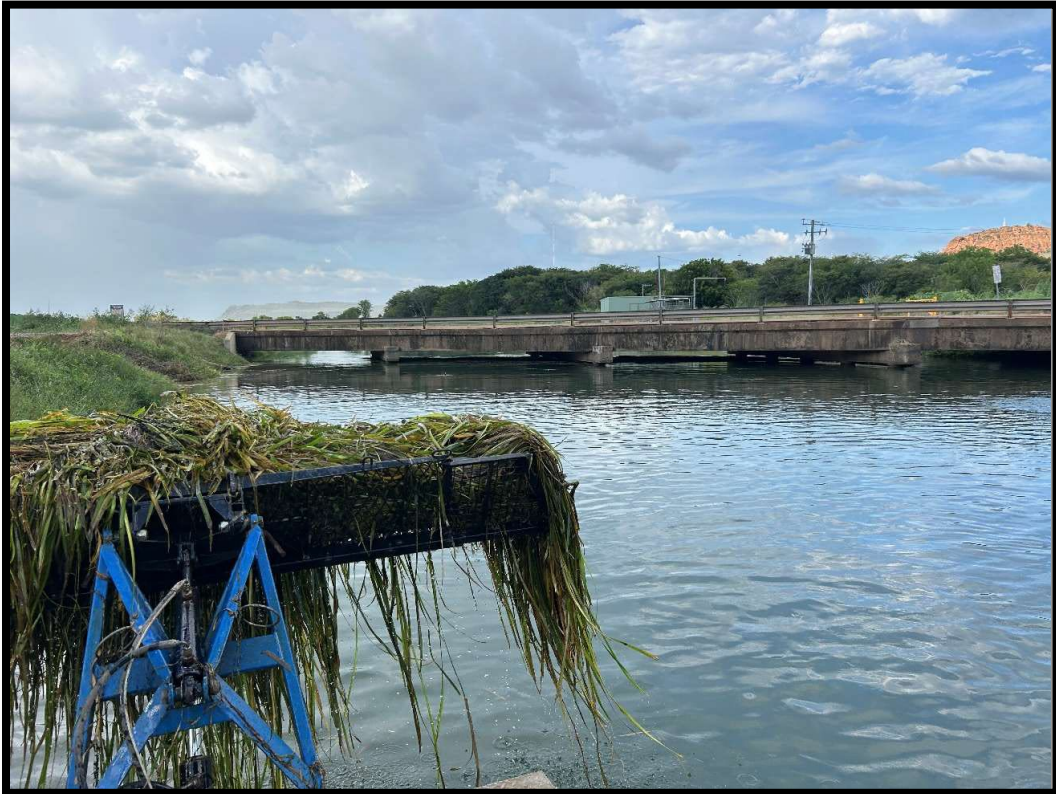
Figure 6: During the removal of weed cuttings in channel - removal of weed cuttings has left minimal weed material in the waterway, improving water quality and flow immediately (Hydroscape Environmental, 2025).
