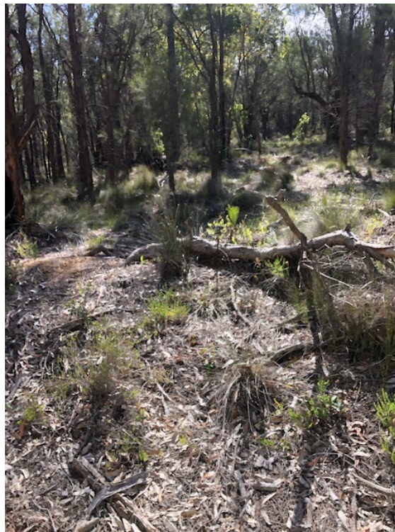
Figure 2 Forest after drilling with a rubber tyre rig
