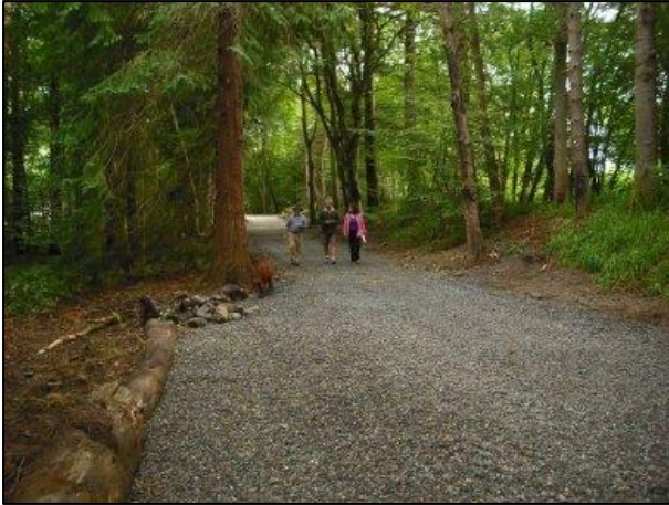
Image 4 – no dig pathway installed over tree roots
