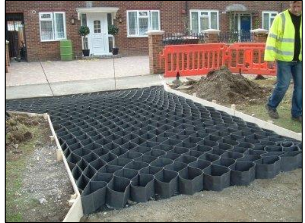
Image 5 – Geocells pre instalment of trafficable material
