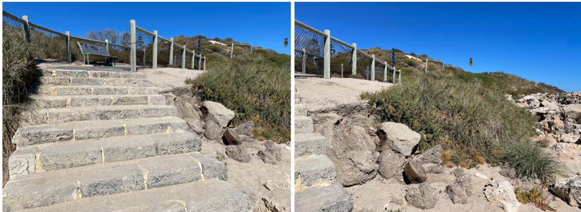
Figure 2.3 Limestone Block Stairs
