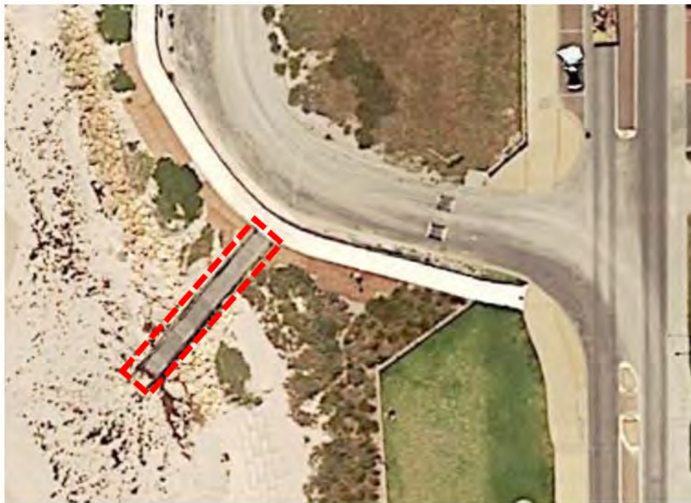
Figure 3.50 C25 Site Inspection Extent
