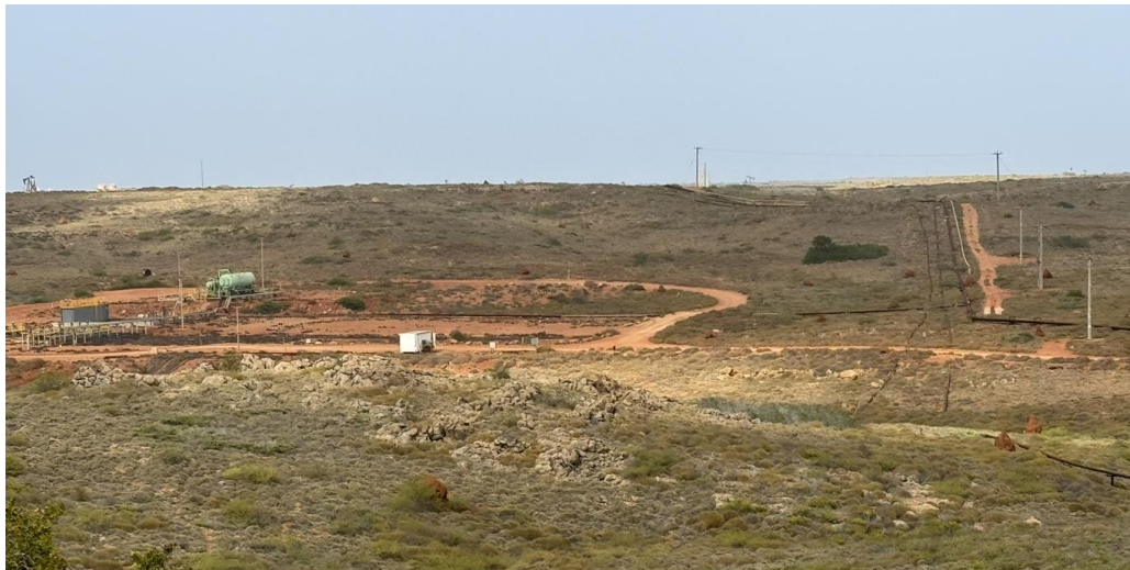
Photograph 3-5: Overhead Power Distribution Network
