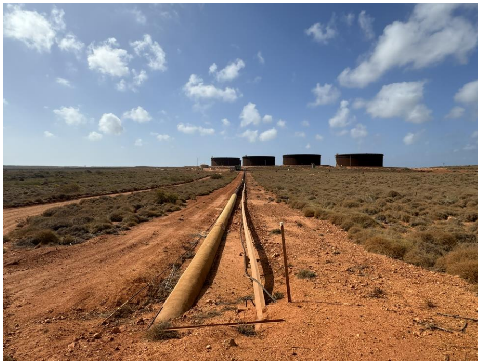
Photograph 3-4: Barrow Tanker Loading Line Onshore Pipeline
