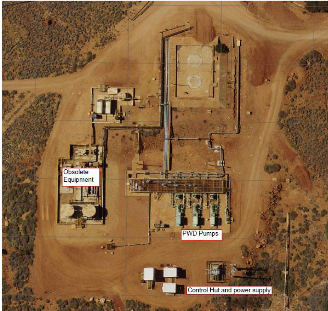
Figure 3-5: Produced Water Disposal Facility
