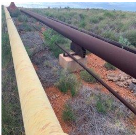
Photograph 3-11: Pipeline (>100 mm) concrete block supports
