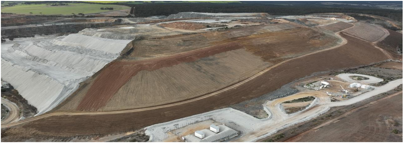
Figure 3. Rehabilitation site preparation (Galaxy Resources Pty Ltd, 2024a)
