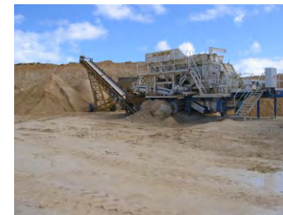
Typical operational crusher
