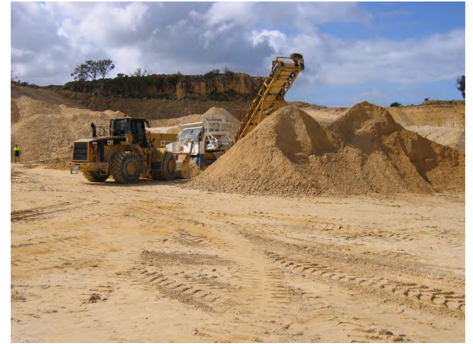
Typical operation on the floor of a quarry with the loader feeding the crusher and small stockpiles
