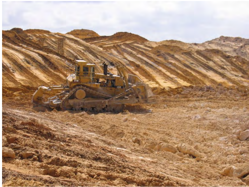
Typical excavation with a bulldozer ripping the limestone
