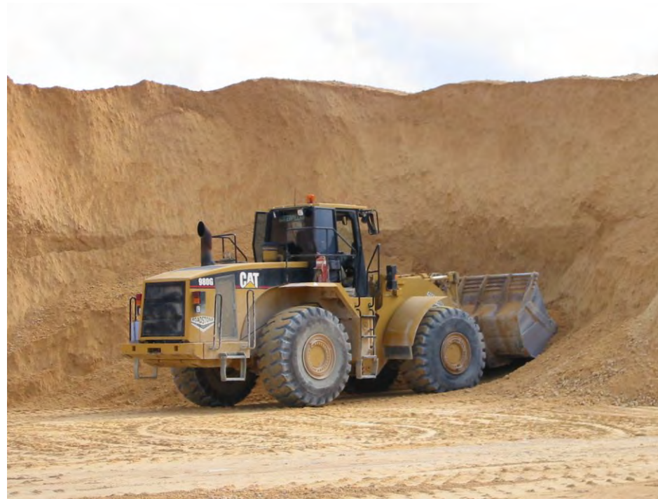
Loader loading screened limestone
