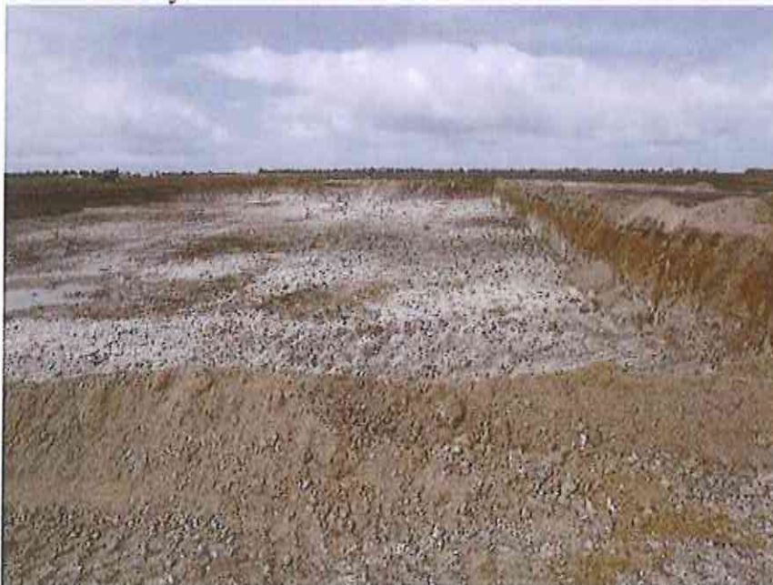
Shallow topsoil and loam over pallid zone clays in main detention basin
