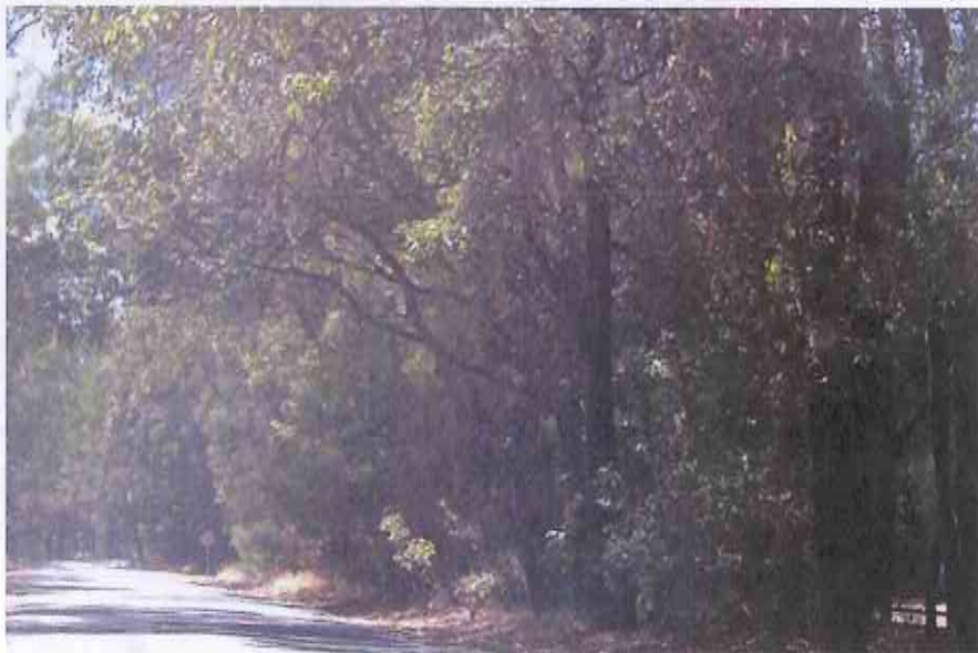
Typical Photo of Road Reserve area - Vasse Yallingup Siding Road, QUEDJINUP
