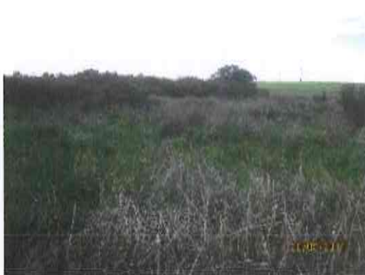
Dam storage area looking to the north east to tee tree which is the limit of the water storage for the dam
