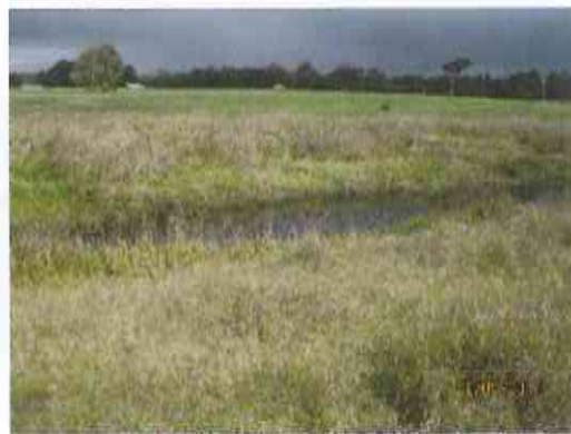
dam storage west area looking to south west
