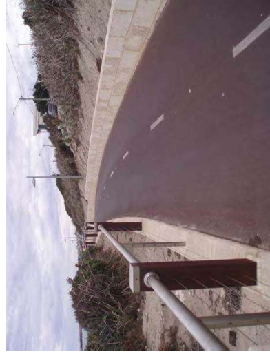
DUAL USE PATH (RED ASPHALT 3m WIDTH)
