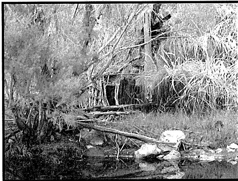
Plate 6: Old Footings of the Bridge
