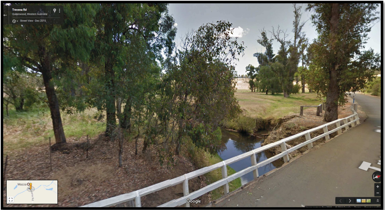
Figure 3. Riparian vegetation, degraded farm land and existing bridge
