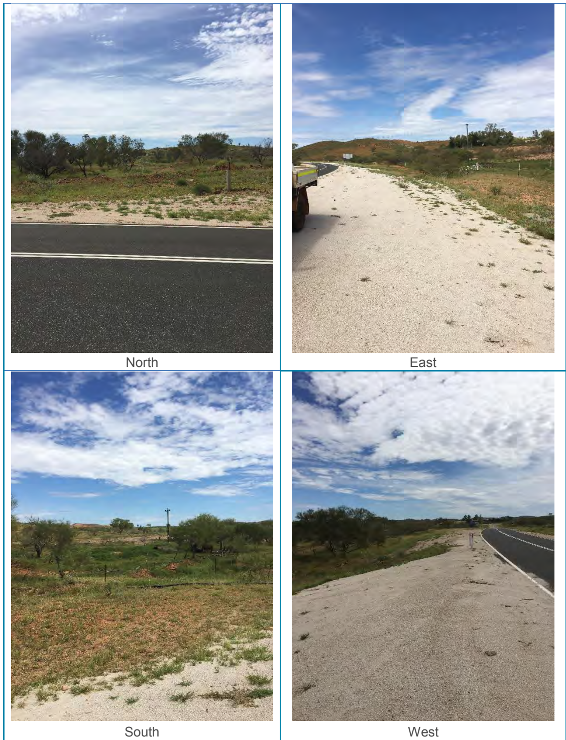
Figure 3: Photo Reference Location 2 - Calcrete
