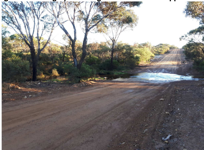
Photo 1: The Western section of the Meechi Road creek crossing will require the removal Eucalyptus occidentalis (flat-topped yate) trees and several small shrubs and sedges.
