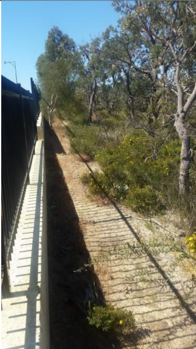
h) Northern boundary to be revegetated, western side of existing stairs (looking east).
