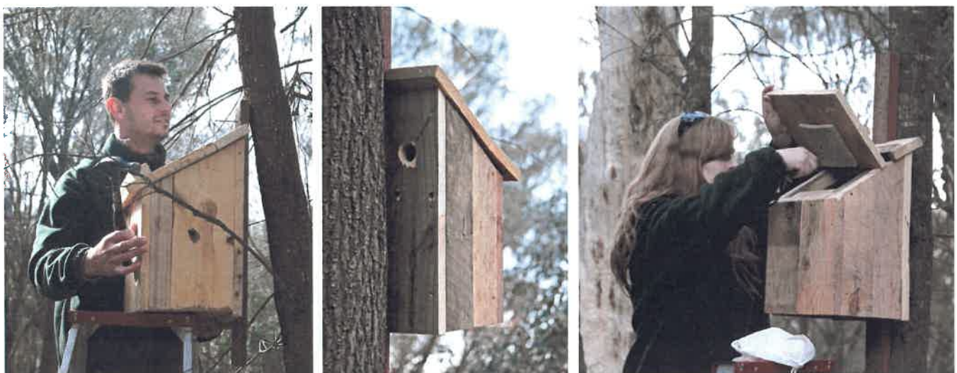
Nest boxes being attached with nails (left), with a rear entrance hole (centre), and with a hinged lid and carpet (right). Photo: Angela Sanders/Bush Heritage Australia (left), DBCA (centre and right)
