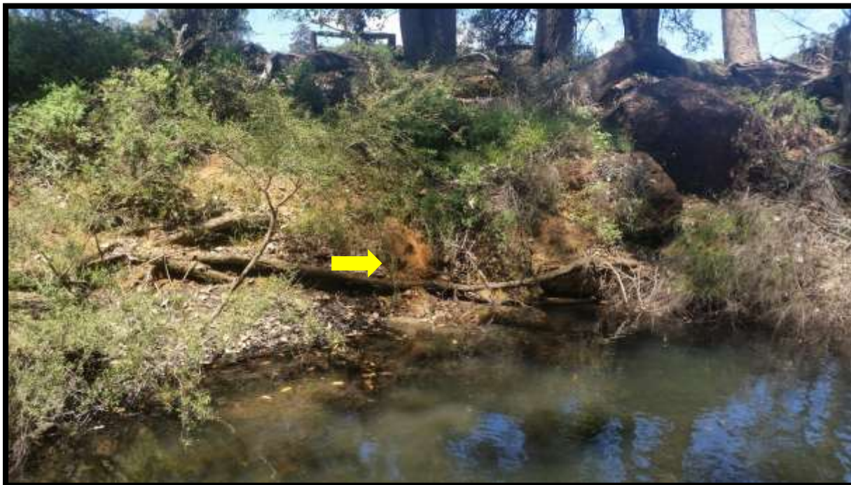
Plate 7: Location 3 - East Bank
