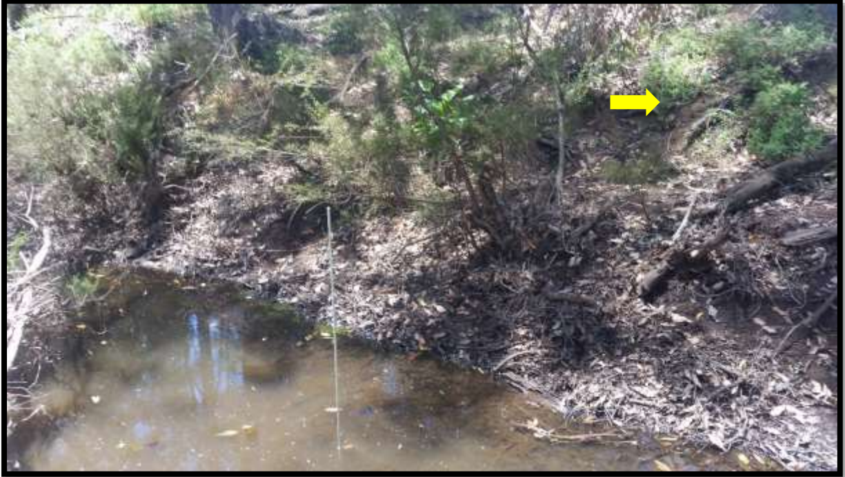
Plate 3: Location 1 – Proposed Bridge/Weir Site - East Bank (Tip of Arrow indicates estimated 59m AHD corresponding to height of weir)
