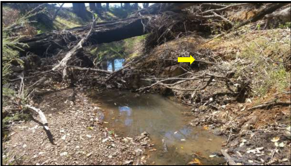
Plate 11: Location 5 - East Bank
