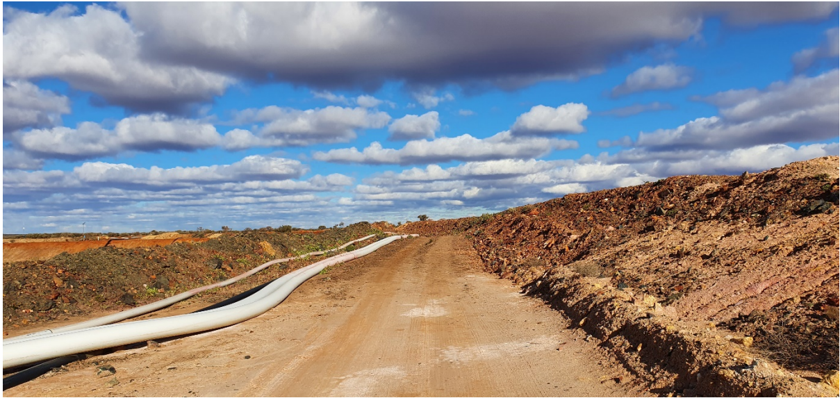
Photo 7. Road South of Pit – Looking South-East
