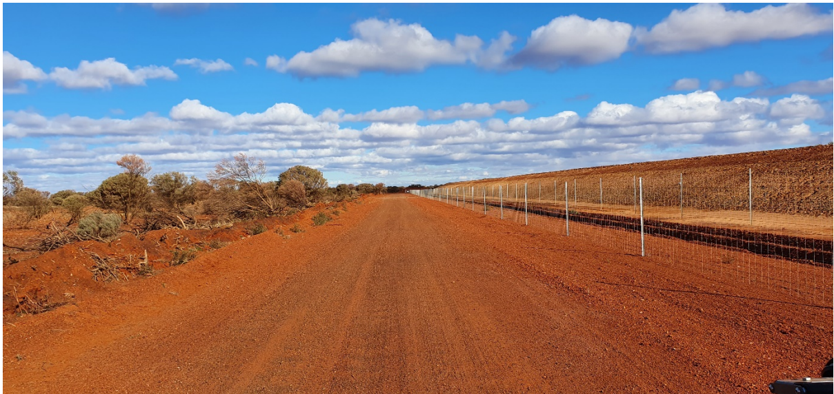
Photo 4. WMP9 (Area 1) – Looking South-South-East
