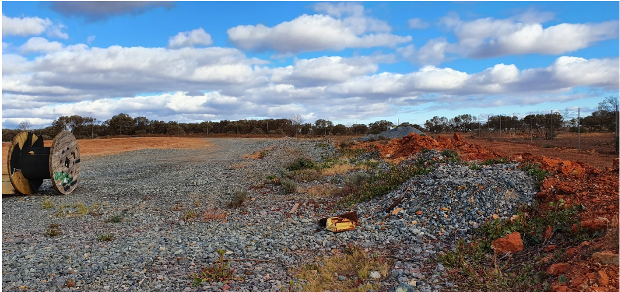
Photo 9. Landfill Facility – Looking South
