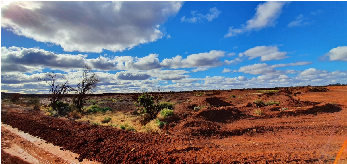
Photo 3. Topsoil (Area 4) – Looking North-North-West
