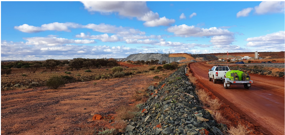
Photo 10. Median North of Fuel Farm – Looking East
