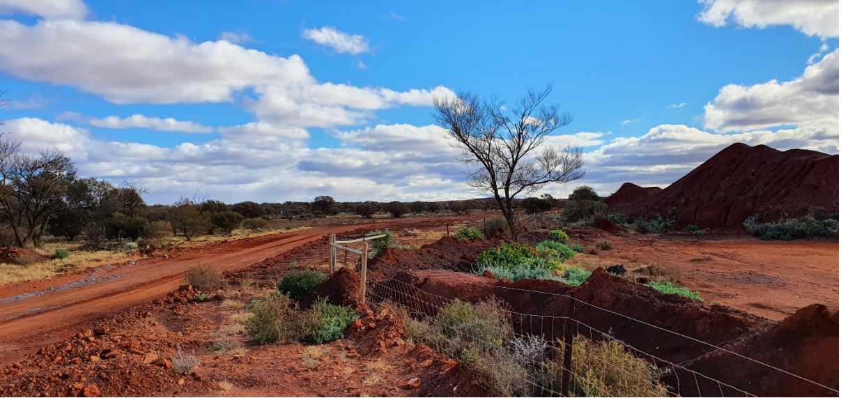
Photo 5. East/West Road to Topsoil/WMP9 – Looking West
