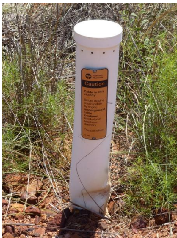
Photo H: Signed underground service spanning entire north-south length along the centre of Site 2.
