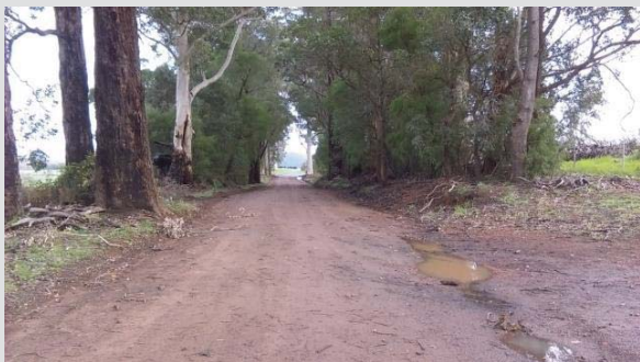
Figure 8: SLK 2.25 looking west
