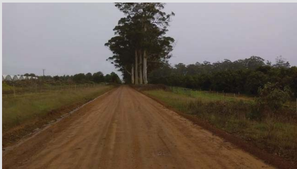
Figure 4: SLK 0.77 looking west
