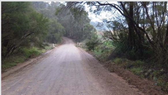
Figure 6: SLK 1.62 looking west towards brook crossing
