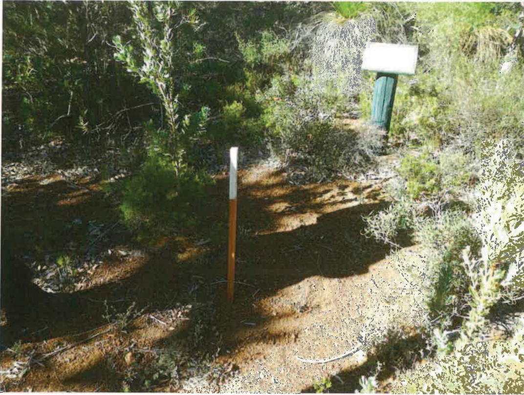
Figure 3: Example of signage installation location for P015. Old infrastructure is being removed but the position of new infrastructure can utilise open areas in order to minimise clearing impacts. The stake with white cap shows the proposed location of P015.
